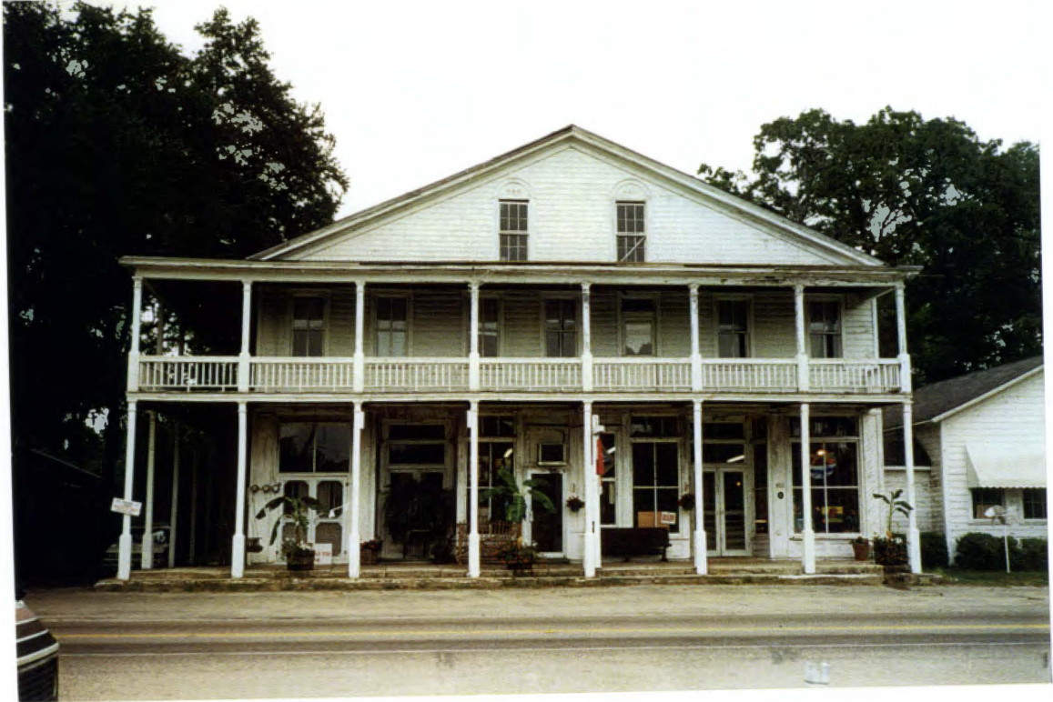
Figure 5.1 The Red Piano Too Art Gallery on St. Helena Island
