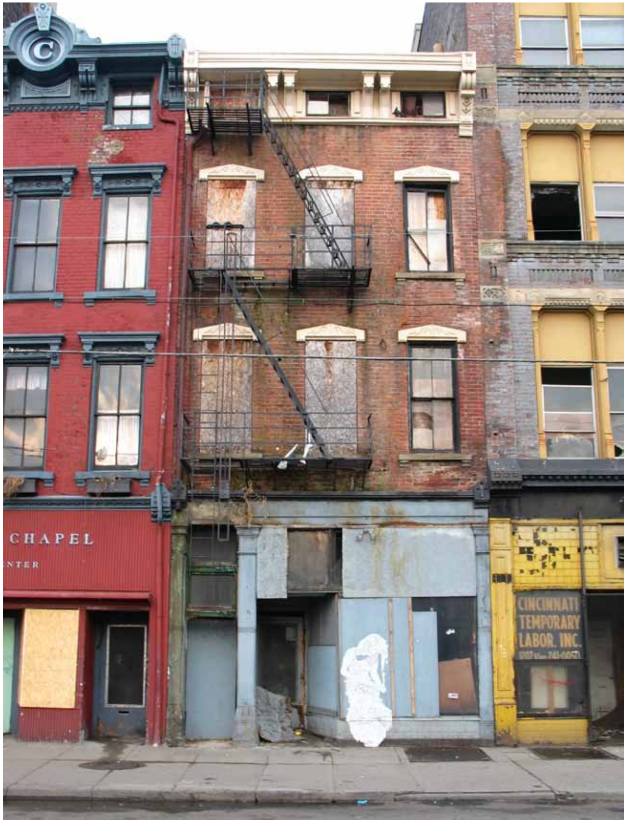
Figure 3: Vacant Building in Over-the-Rhine
