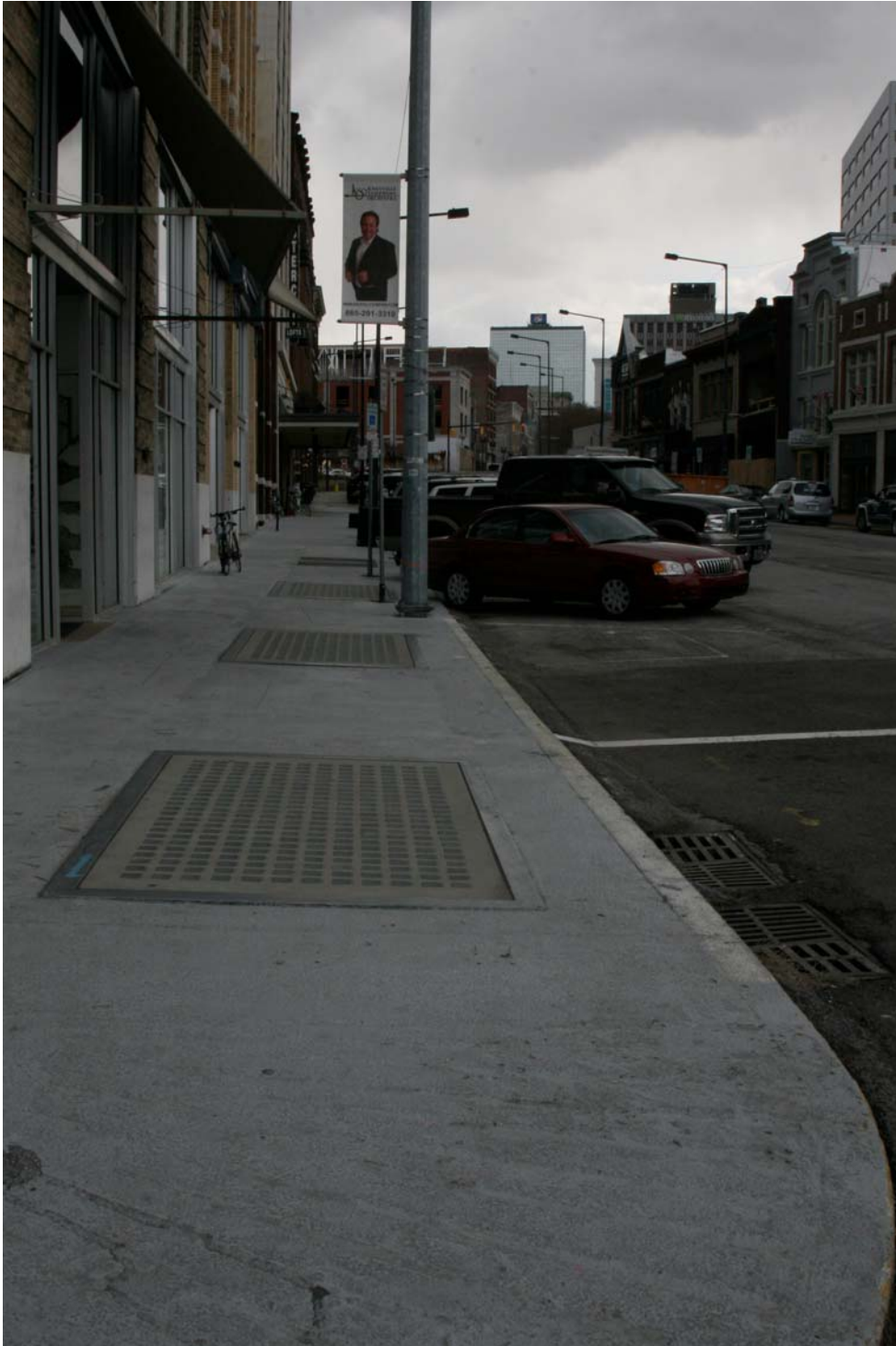
Figure 13: 100 Block of Gay Street looking south; showing the glass tile sidewalk that hints at Underground Knoxville below. Image: Author
