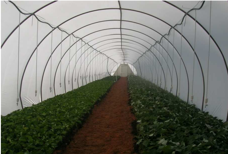
Figure 3-3. Polyhouse covered groundbed system (photo courtesy of Dr. Charles Hall)
