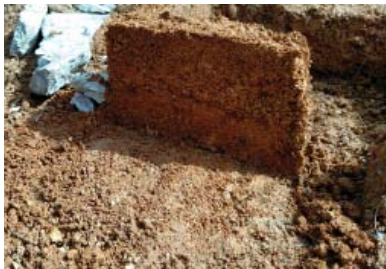
Figure 73: In Situ - Wall
