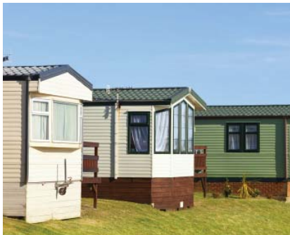
Figure 33: Mobile Homes. These were likely built completely in a factory and delivered as one unit to the site.
