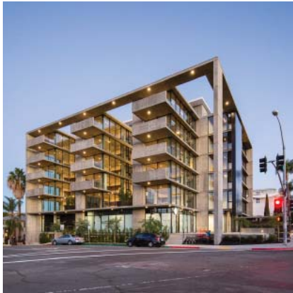
Figure 20: Mr. Robinson Housing Development. San Diego, CA.
