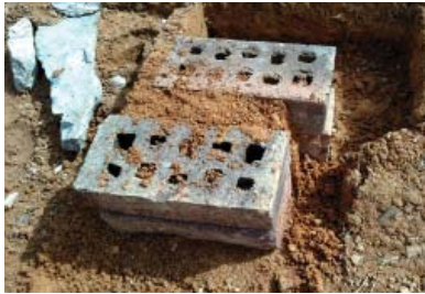
Figure 72: In Situ - Wall Forms
