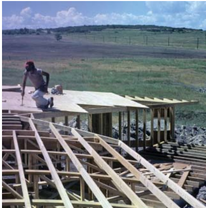
Figure 21: Constructing the Airplane House
