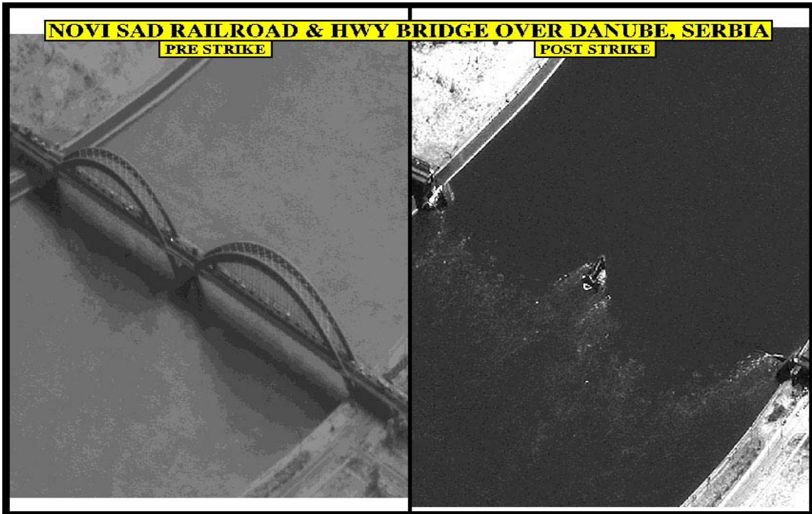
Figure 2-2 (DOD photograph) Zezeljev Bridge during Kosovo War Before and After JDAM Attack
