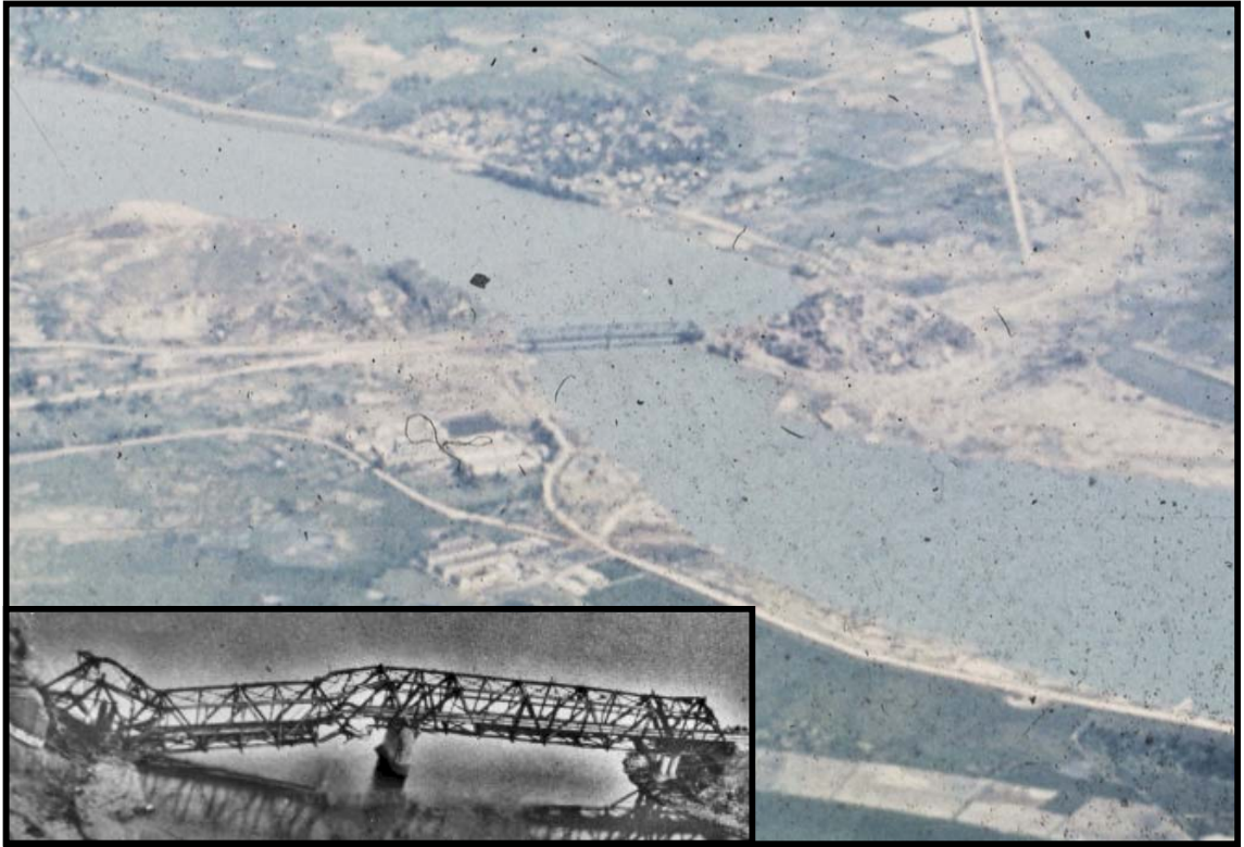
Figure 2-1 [6], [7 inset] Thanh Hoa Bridge, Vietnam Pre-Strike and Post-Strike (inset)
