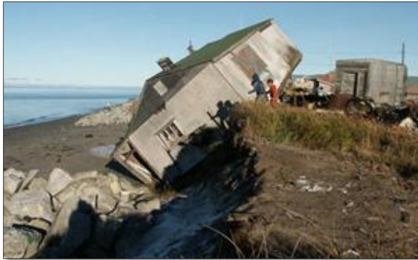
Figure 15 House in the Alaska Native village of Shismaref (Alaska Conservation Foundation 2010).
