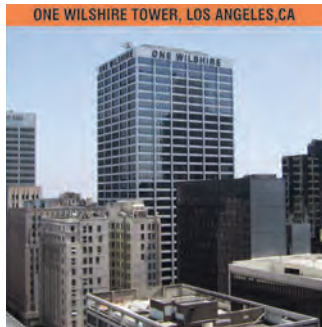
Figure 9: One Wilshire Tower
