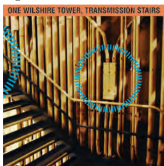
Figure 15: One Wilshire Tower
