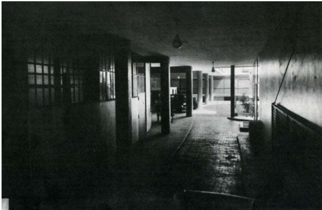
Figure 2 – Secondary entrance corridor Cite de Refuge
