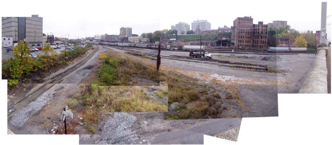
Figures 29- L & N Railroad yard looking toward downtown Photo by author
