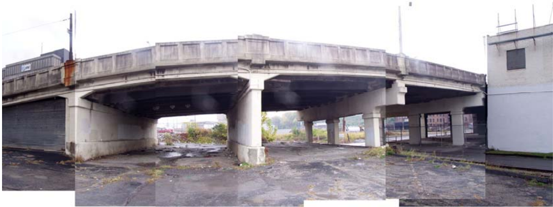
Figure 21 –Below Broadway Avenue bridge Photo by author
