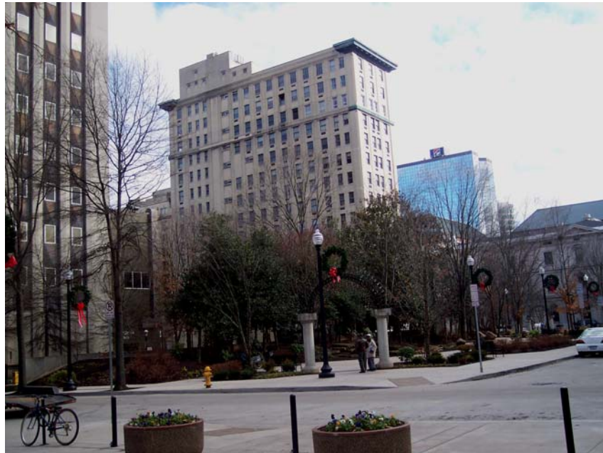
Fig. 2.8: View of Site from Market Square Source: Author
