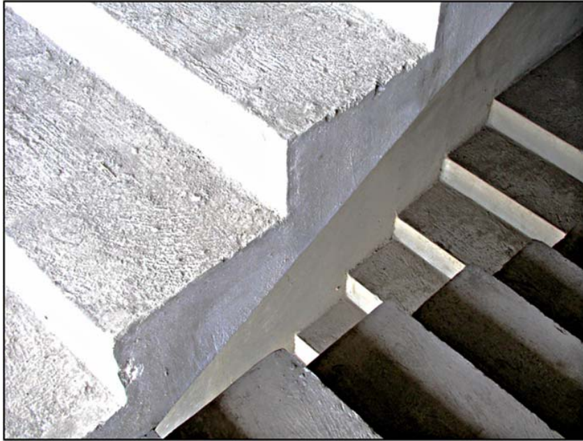
Fig. 2.3: Concrete Stairway Source: Challenging Technologies, LLC
