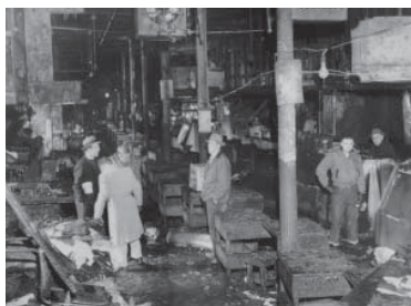
Figure 016 Workers evaluate the Market Hall after the fire, but before demolition. Many thought that the Market Hall could be salvaged and repaired, but demolition continued contrary to public outcry.
