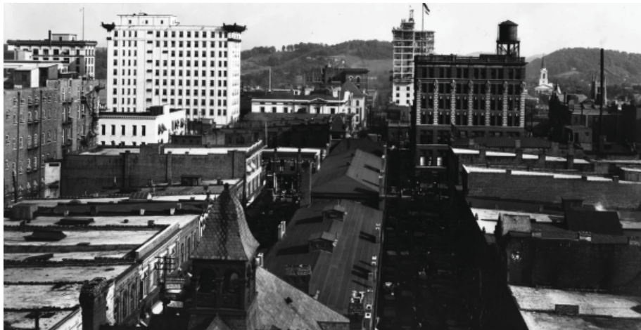
Figure 007 View of the Market Hall roof, facing south.
