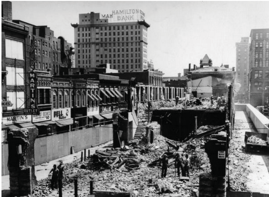
Figure 015 Exterior photograph of the Market Square Market Hall after the fire and demolition.
