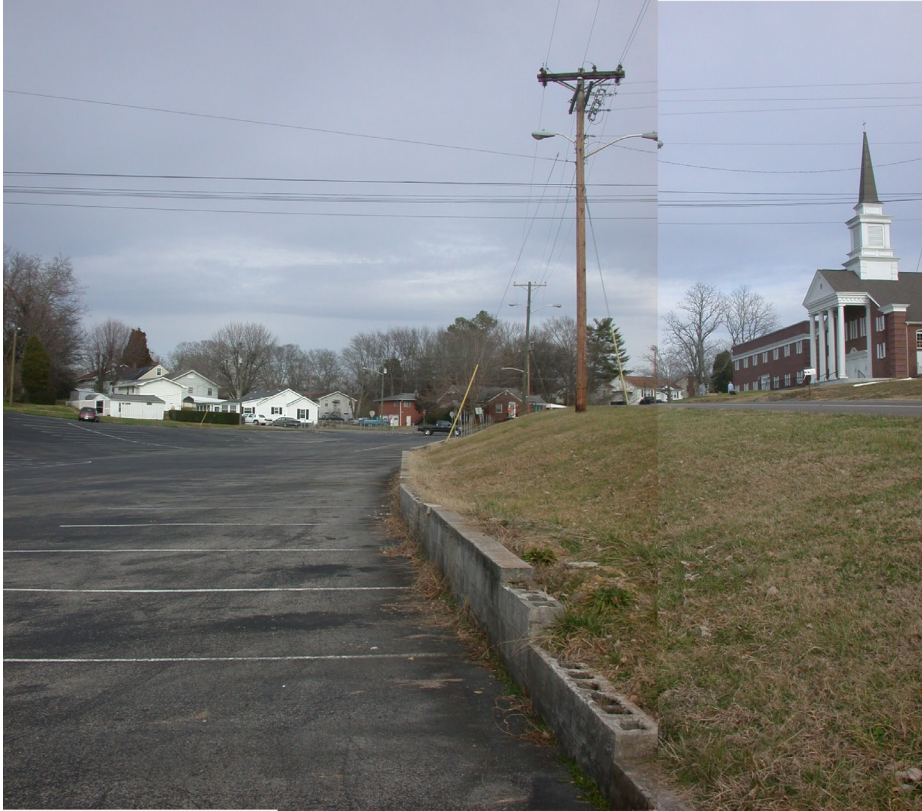
55. Looking along existing retaining wall. SOURCE: author, Jan. 2007
