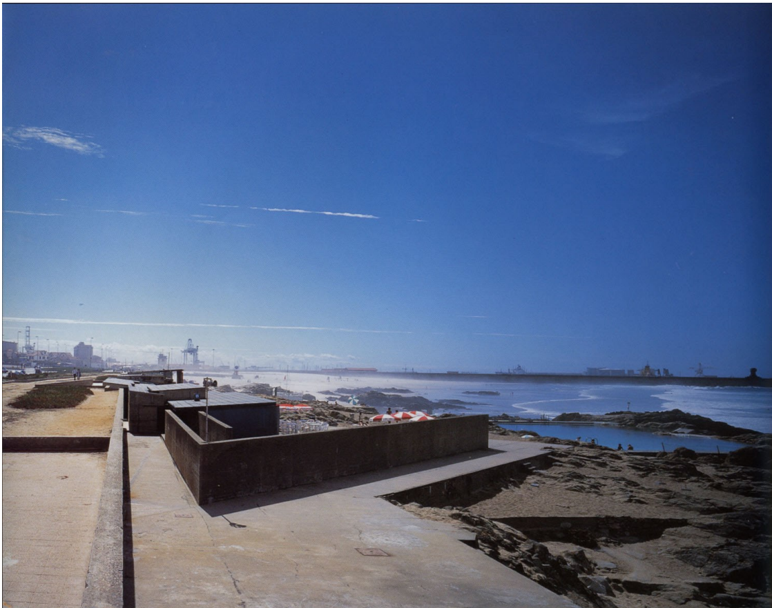
28. View with industrial area beyond, looking south. SOURCE: Luiz Trigueiros
