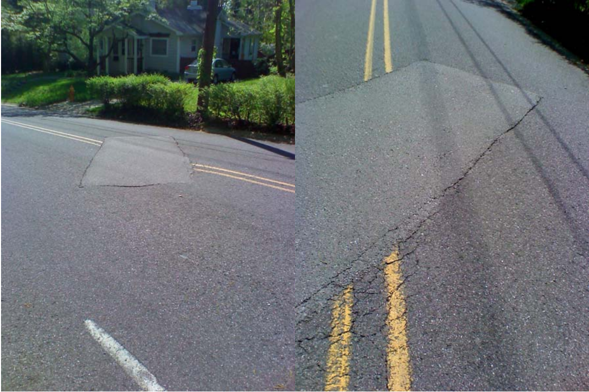
Figure 100 – Photographs – 165 California Avenue, COR
