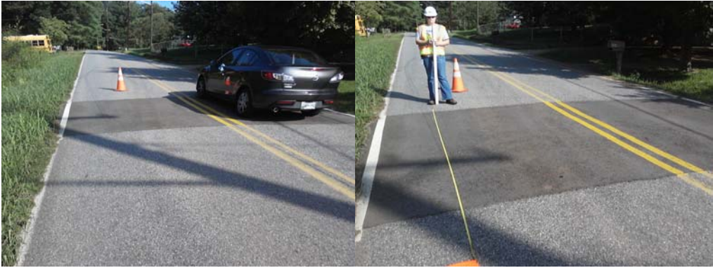
Figure 155 – Photographs – 204 Stone Road, KUB
