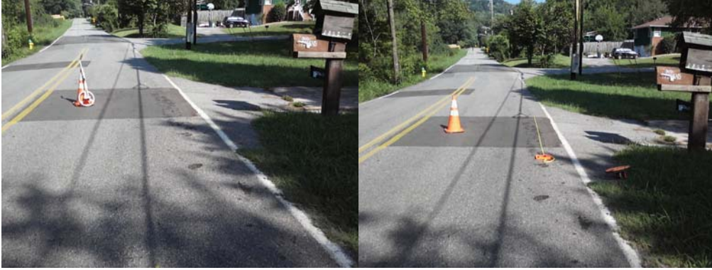
Figure 161 – Photographs – 300 Stone Road, KUB
