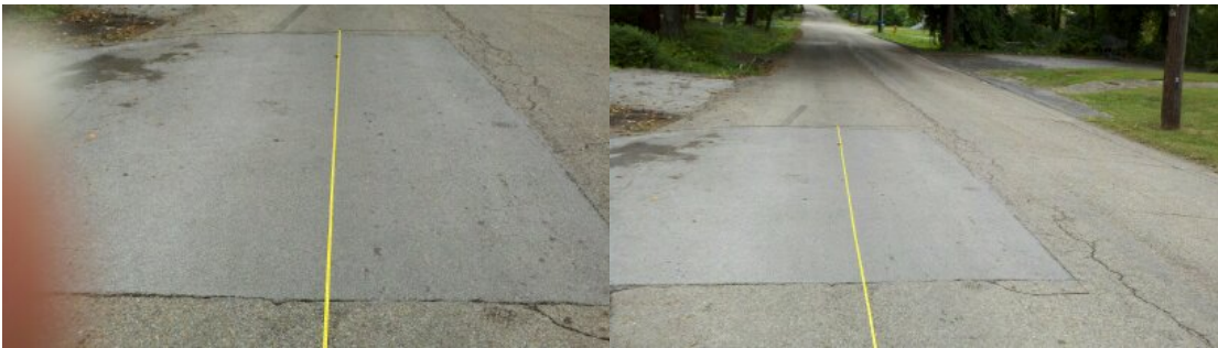
Figure 128 – Photographs – 3111 Rennoc Road, KUB
