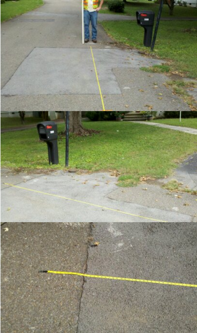
Figure 140 – Photographs – 5028 Hedgewood Drive, KUB
