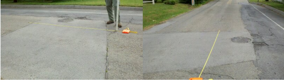
Figure 119 – Photographs – 2857 Rennoc Road, KUB
