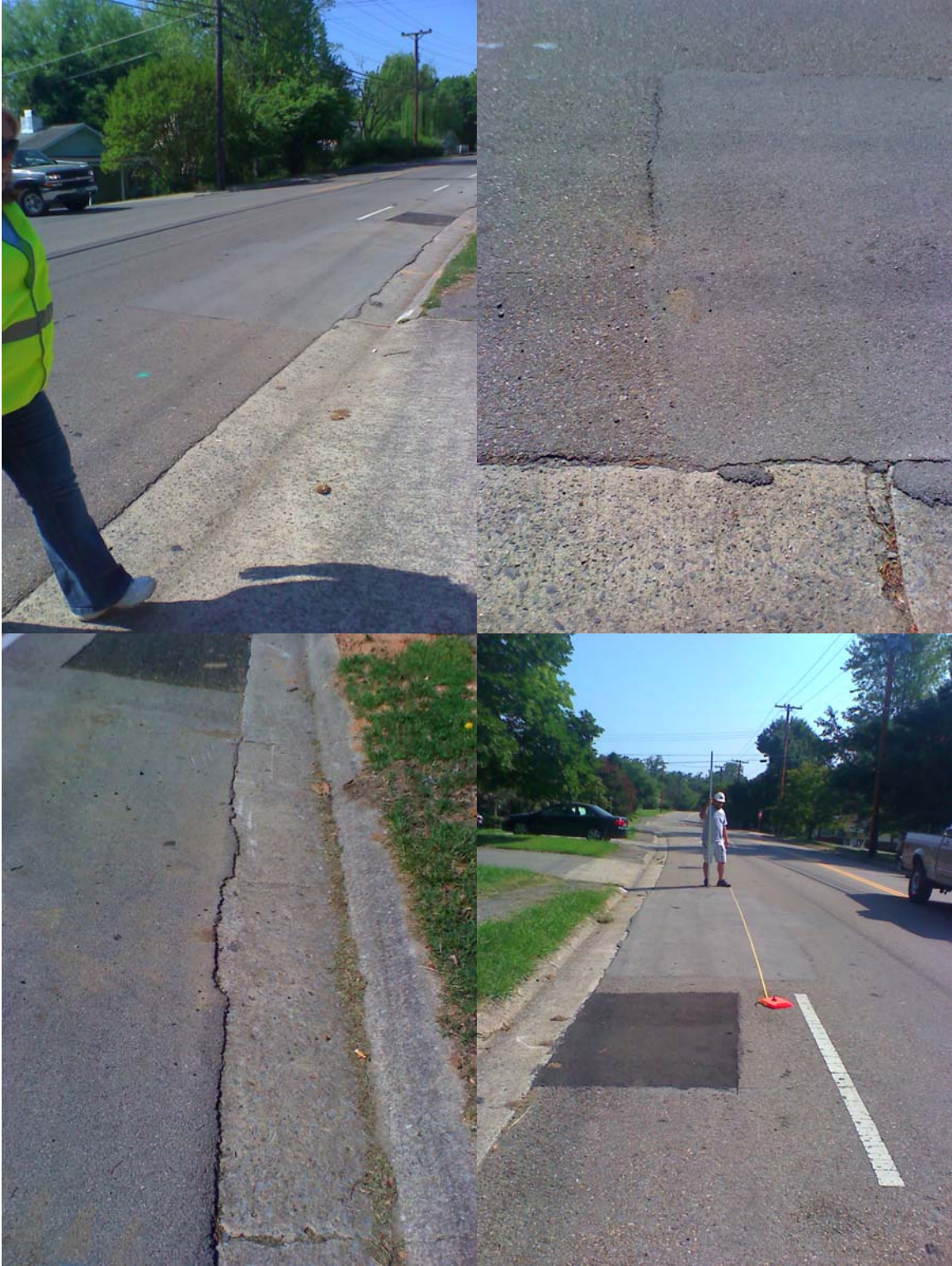
Figure 109 – Photographs – 309 East Tennessee Avenue, COR
