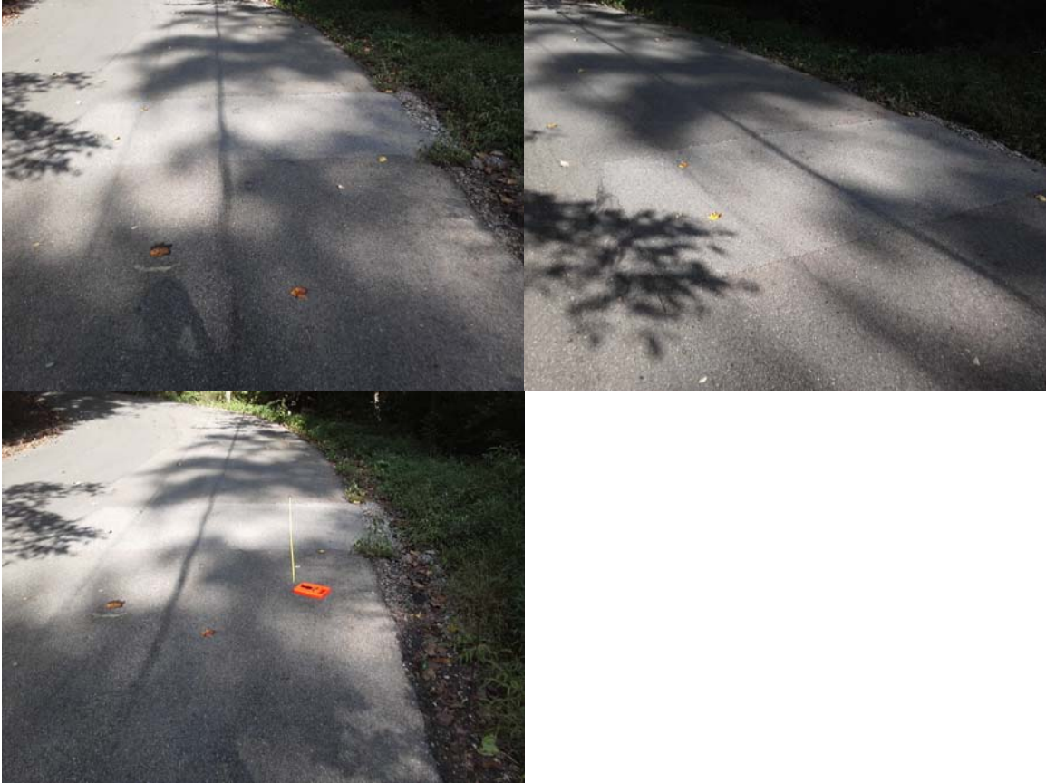
Figure 178 – Photographs – Wise Hills Road, KUB
