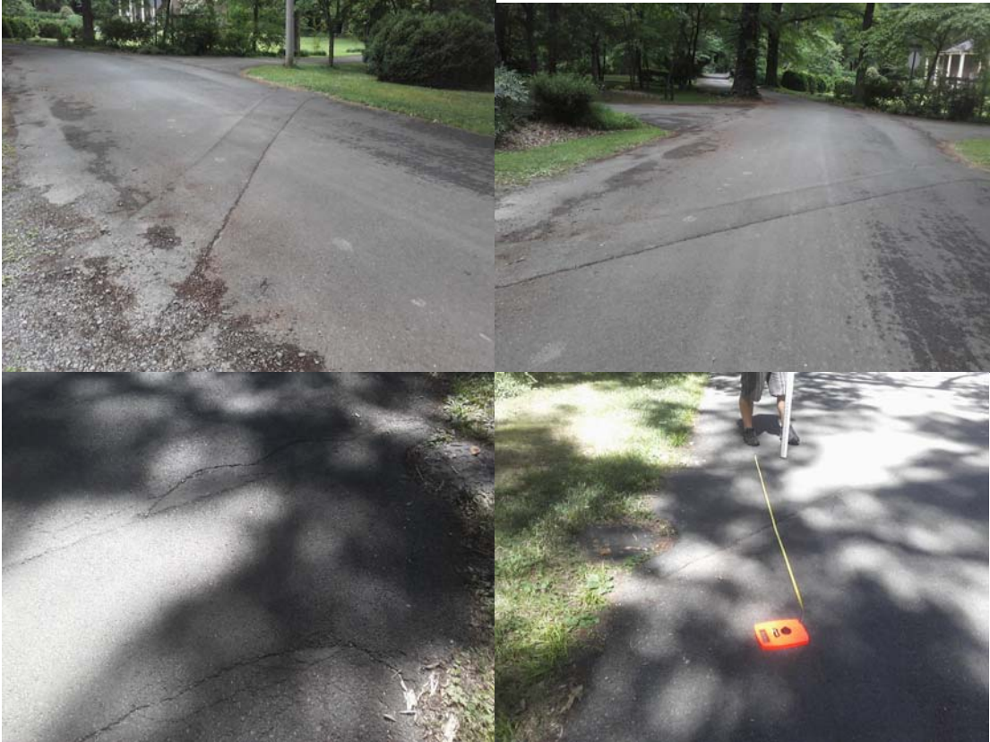
Figure 42 – Photographs – 605 Getty's Lane, AUB
