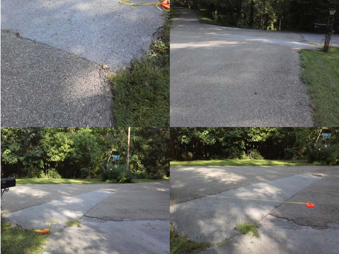
Figure 158 – Photographs – 220 Wise Hills Road, KUB
