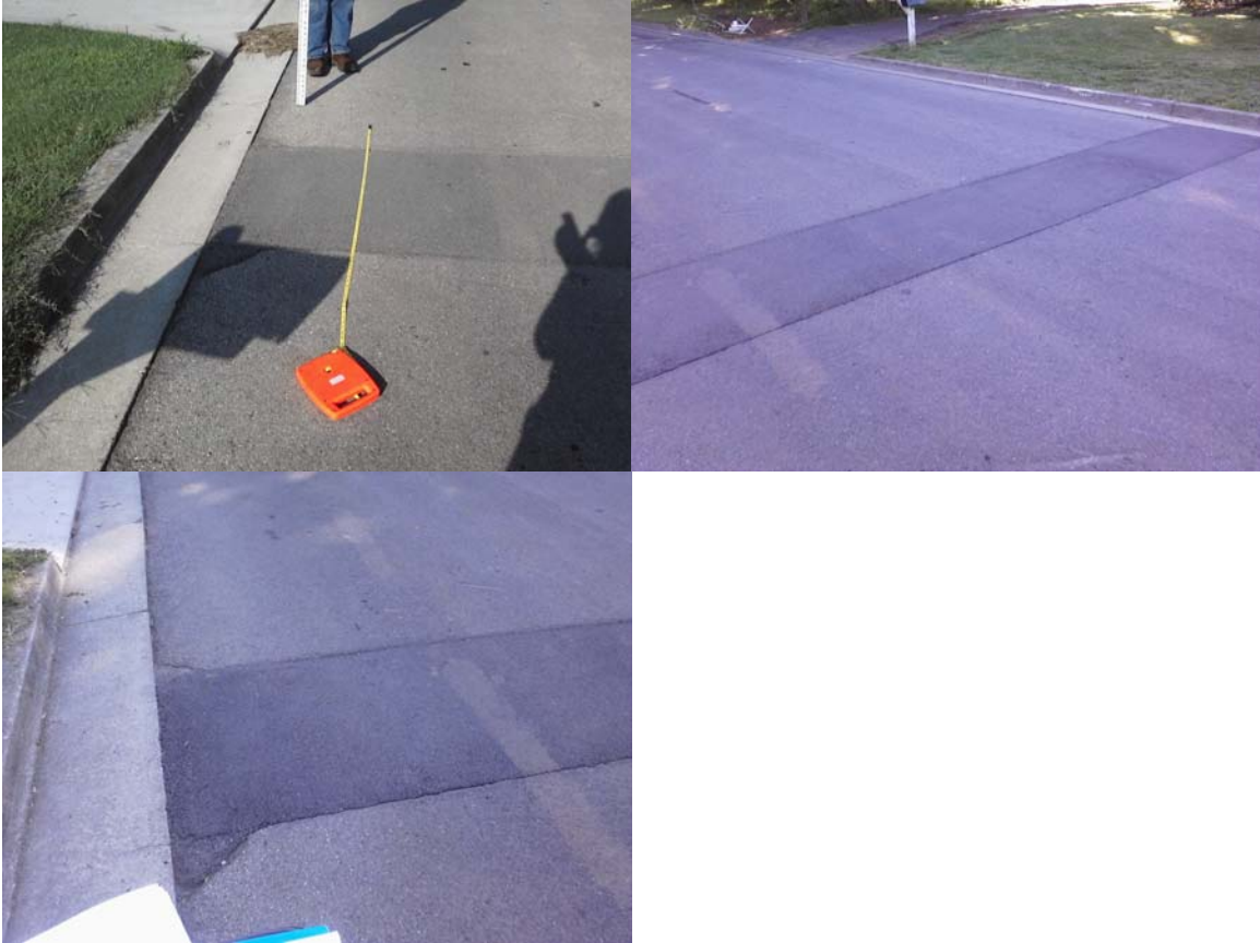
Figure 76 – Photographs – 1107 Everett Avenue, COM
