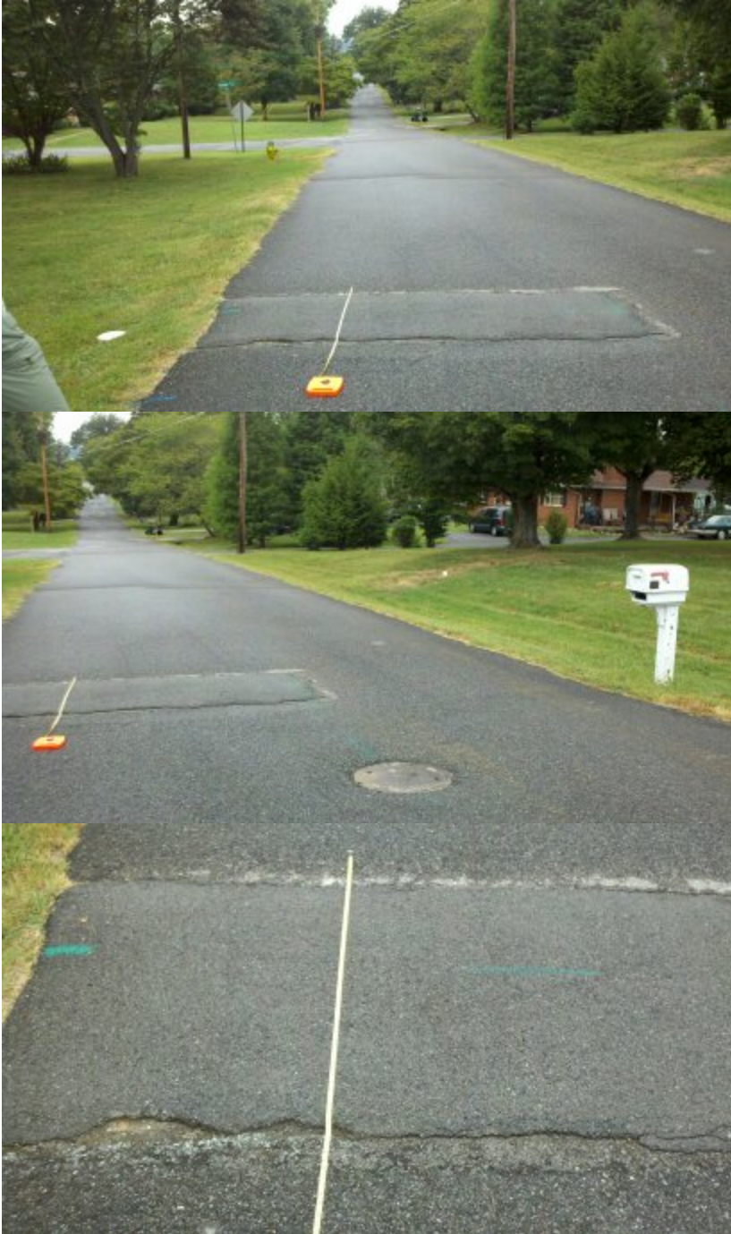
Figure 166 – Photographs – 501 Tedlo Lane, KUB
