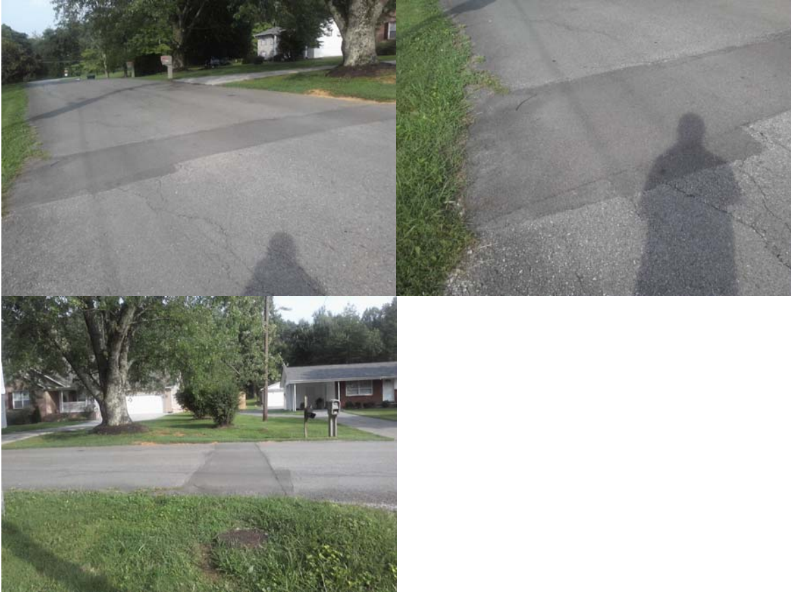
Figure 184 – Photographs – 7913 Wieblo Drive, WKUD
