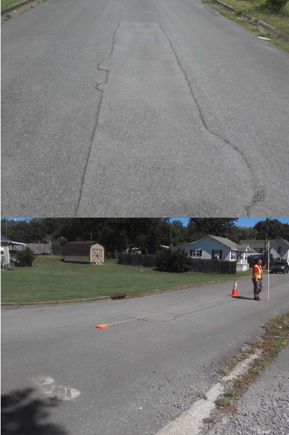
Figure 30 – Photographs – 302 Dixon Avenue, AUB
