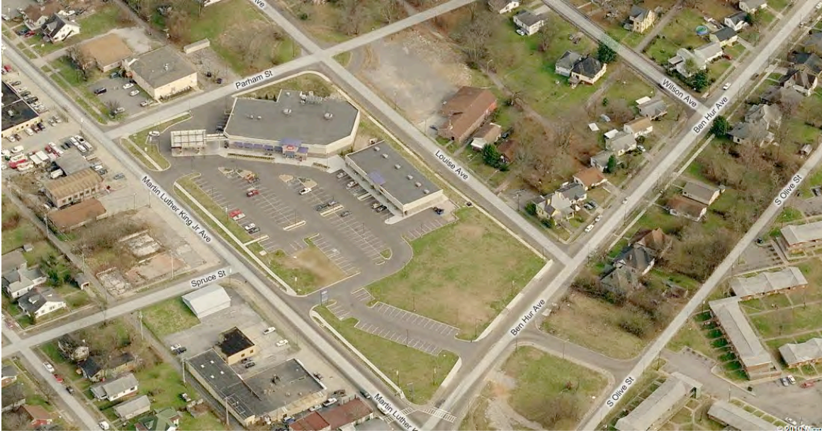
Figure 20. Bird's Eye View of site with old Metro Village Market building. ( www.bing.com/maps ).
