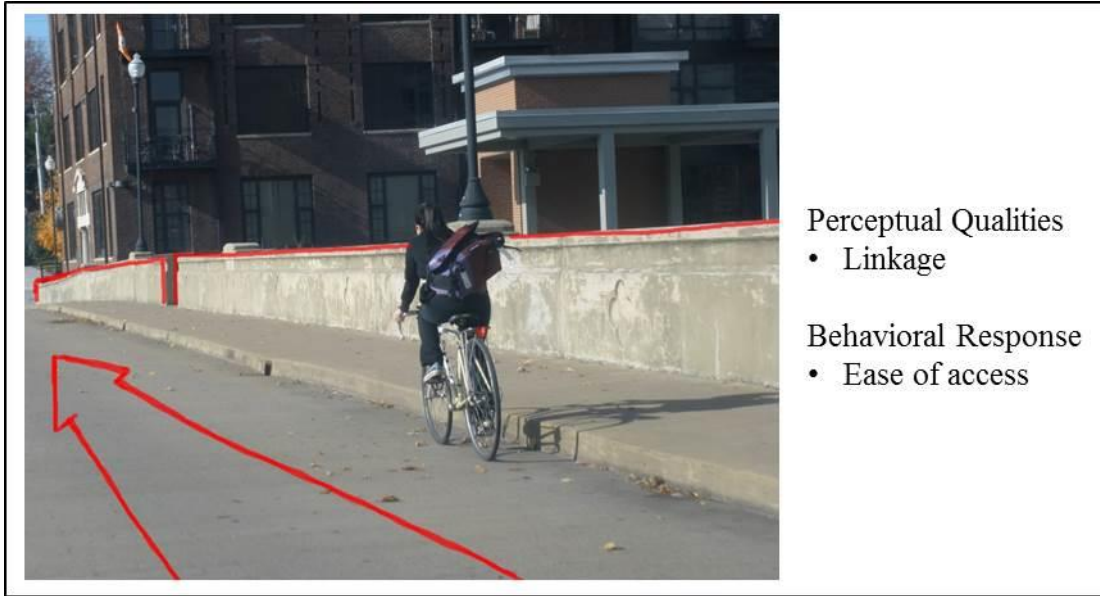
Figure D.55: (c) – Linkage / Ease of access Clinch Ave. Bridge creates a connection between Downtown Knoxville and Fort Sanders and UT campus.
