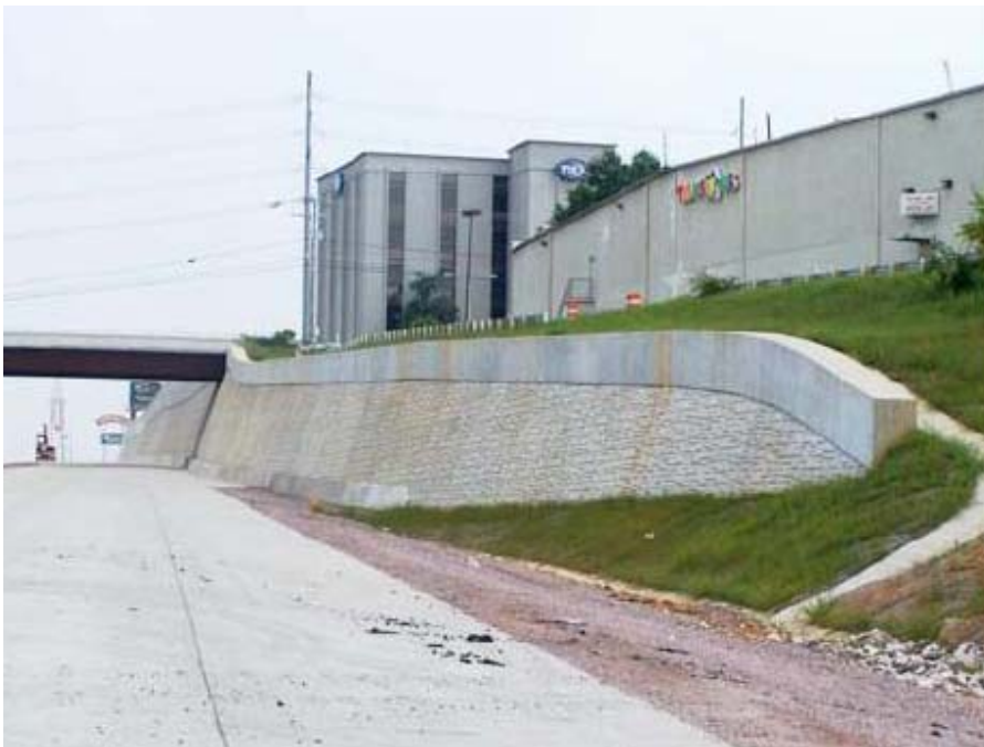
Figure 1.1-1 Completed Pile Framed Wall (Pate and Haddad, 2007)
