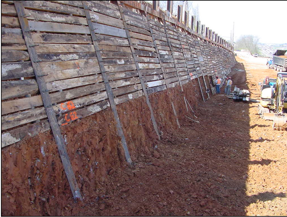
Figure 3.4-1 Construction Photo of Wood Lagging (Courtesy of Saieb Haddad)
