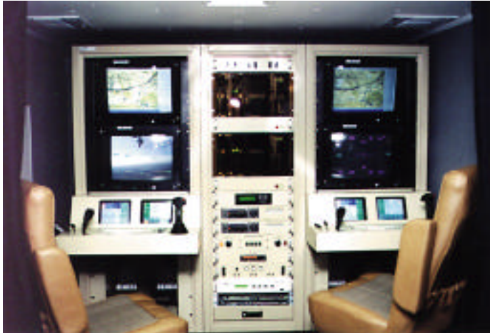
Figure 2-3. Predator Ground Control Station
