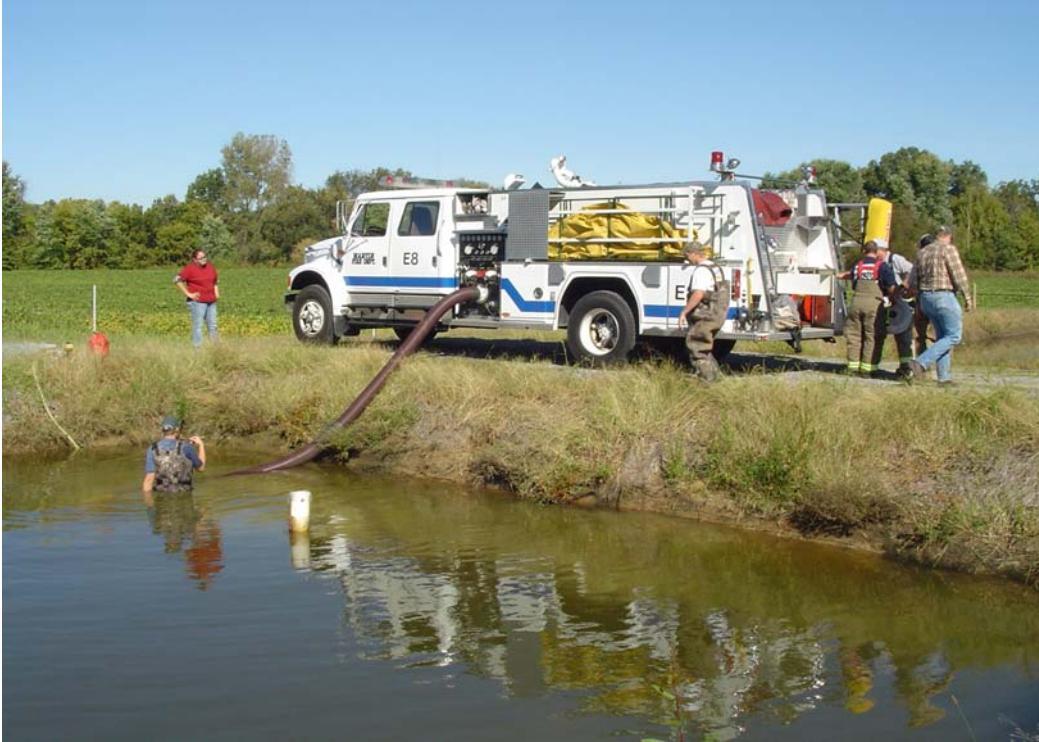
Figure 10. Water was pumped out of ponds at the UT Martin site due to inefficient draining.
