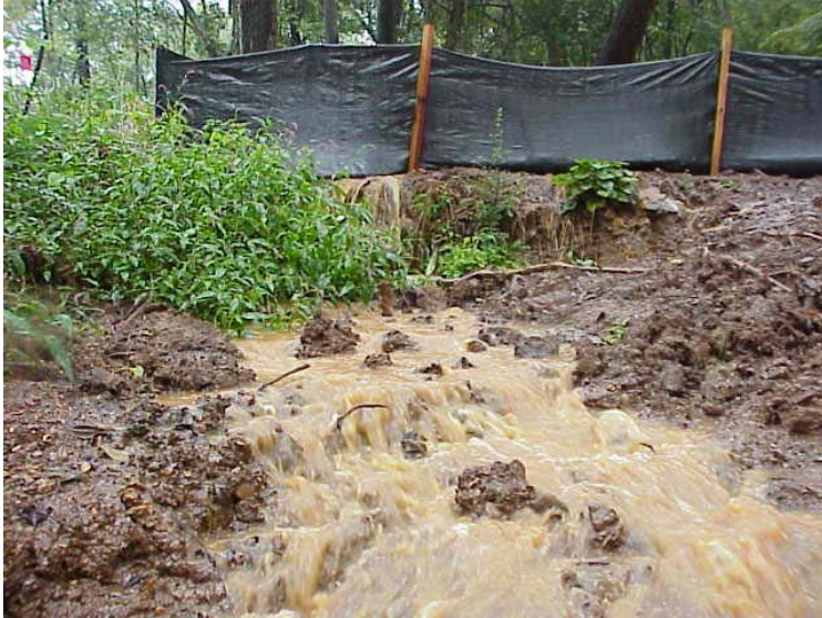
Figure 2. Construction site runoff. April 10, 2004; Wee Williams Golf Course, Knoxville, TN.
