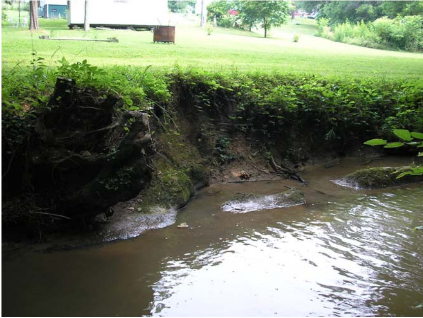
Figure 1. Denuded stream bank. June 22, 2005; Site14, Hines Branch.
