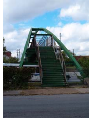
04:04-05 A.) Pedestrian Bridge Over I-40 (Photos by author)
