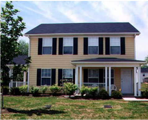
03:04 Vine Hill Homes 2 (Hope VI) (Photo courtesy of Sherman/Carter/Barnhardt Architects)
