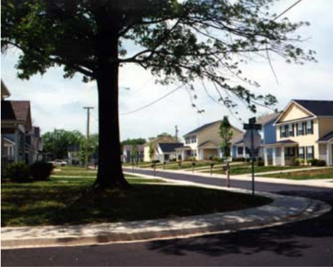
03:03 Vine Hill Homes 1 (Hope VI) (Photo courtesy of Sherman/Carter/Barnhardt Architects)
