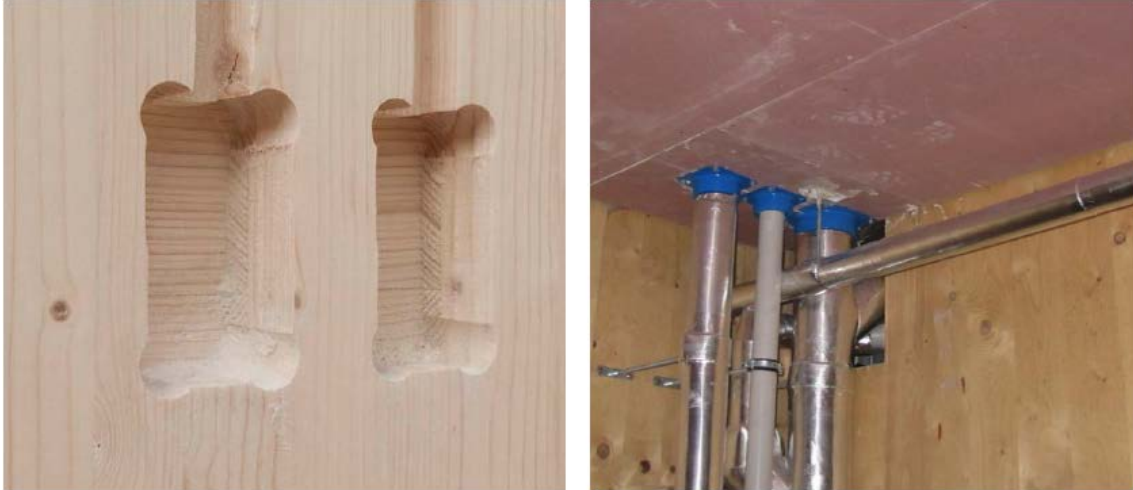
Figure 22: Matchings on pre-fabricated panels (Lend Lease, 2013). Courtesy of Lend Lease
