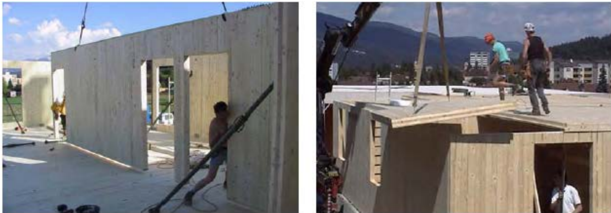
Figure 9: Images of platform construction (Augustin, 2008). Courtesy of Institute of Timber Engineering and Wood Technology, TU Graz
