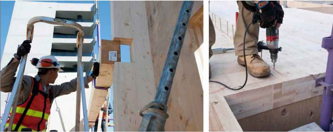
Figure 19: Construction work 'Forté' (Lend Lease, 2013). Courtesy of Lend Lease
