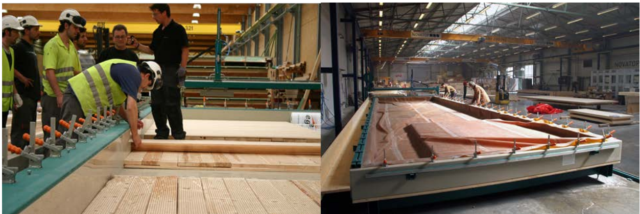
Figure 30: CLT layup in vacuum press (right) sealing with vacuum sheet (right). Courtesy of Woodtec Fankhauser
