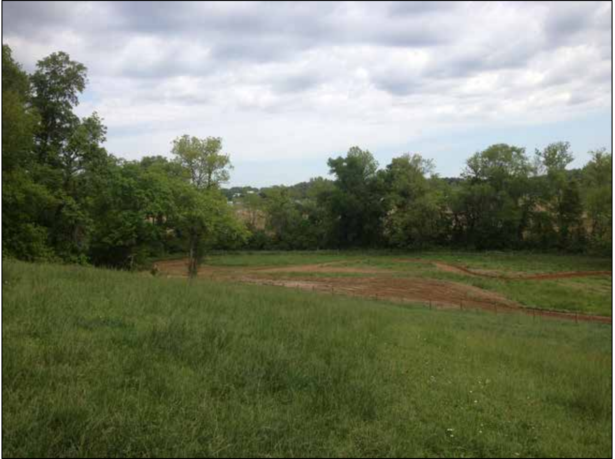
Figure 2.13 A second constructed wetland was installed in Pasture 1 (see Figure 2.4 for location) based on knowledge of groundwater flow directions from the dairy into Pasture 1. Pasture 1 borders Ellejoy Creek to the east. The configuration of the wetland allows for catchment of stormwater runoff as well as flow from an ephemeral stream that borders Pit 1. (Ludwig, 2011).
