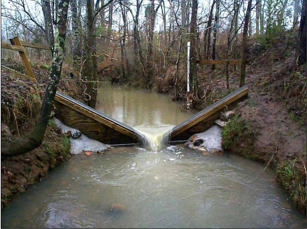
Figure 2.7 - Farm Stream (FS-2) -120 degree V-notch weir.
