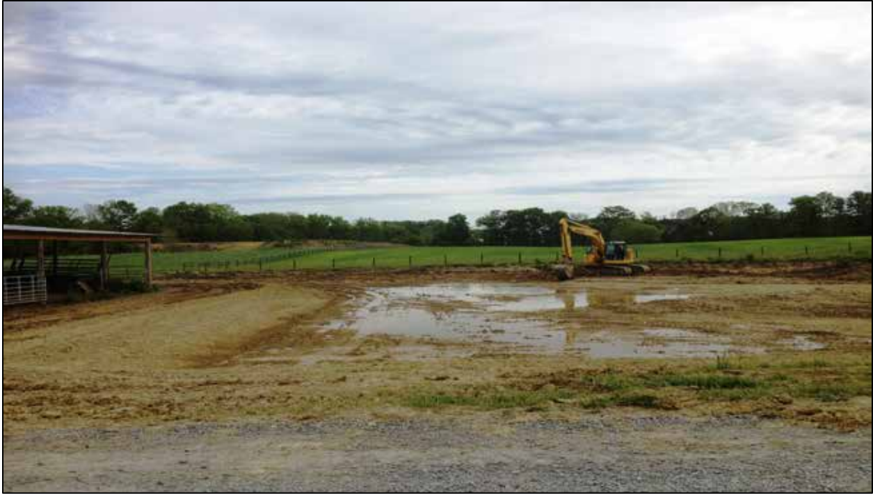
Figure 2.10 Constructed wetland underway (Ludwig, 2011).
