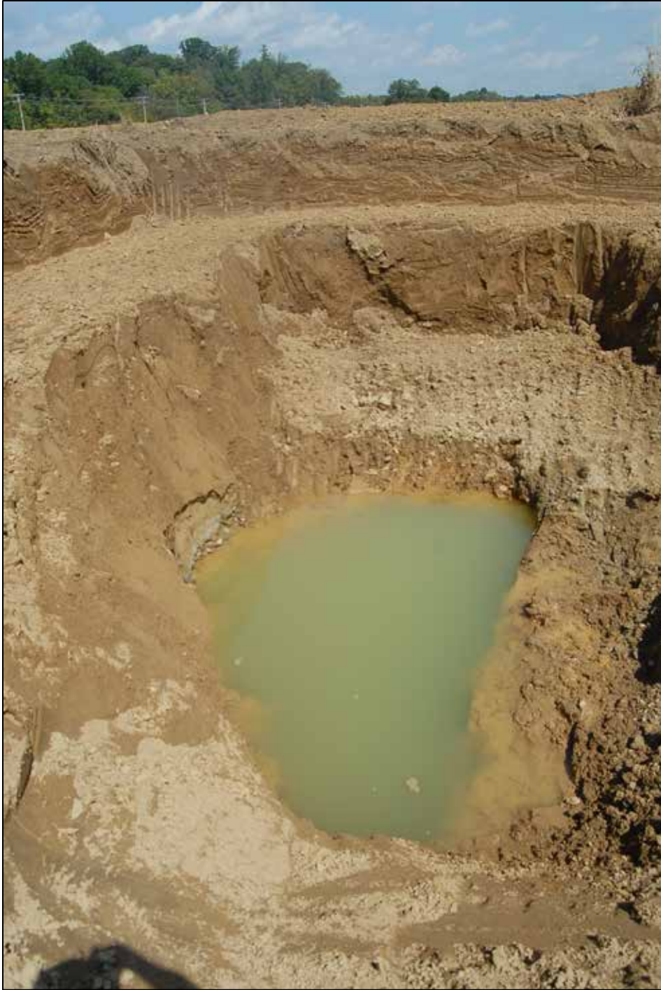
Figure 3.18 – Sinkhole excavation near Well 9 before backfilling with shot rock. Bedrock (right side) was exposed and measured below the water level. The bedrock contains an open cavity dipping toward the southwest below the waterline.
