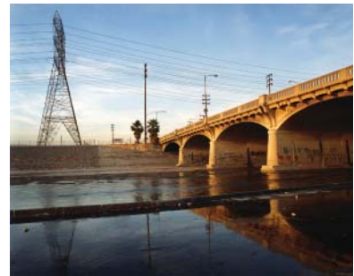
Figure 15: Atlantic Blvd. Bridge, photo 1
