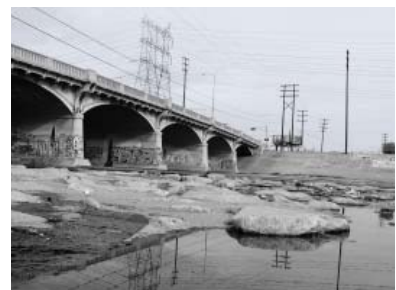
Figure 17: Atlantic Blvd. Bridge, photo 3
