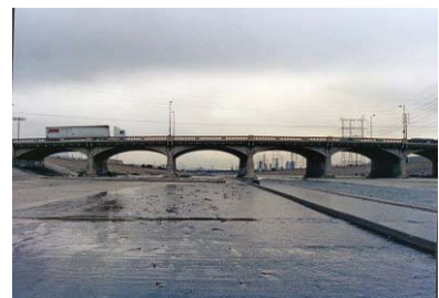
Figure 16: Atlantic Blvd. Bridge, photo 2
