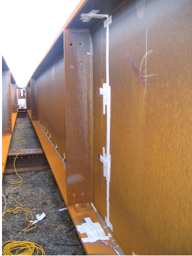
Figure A8: Photograph of Strain Gages and Wires After Installation
