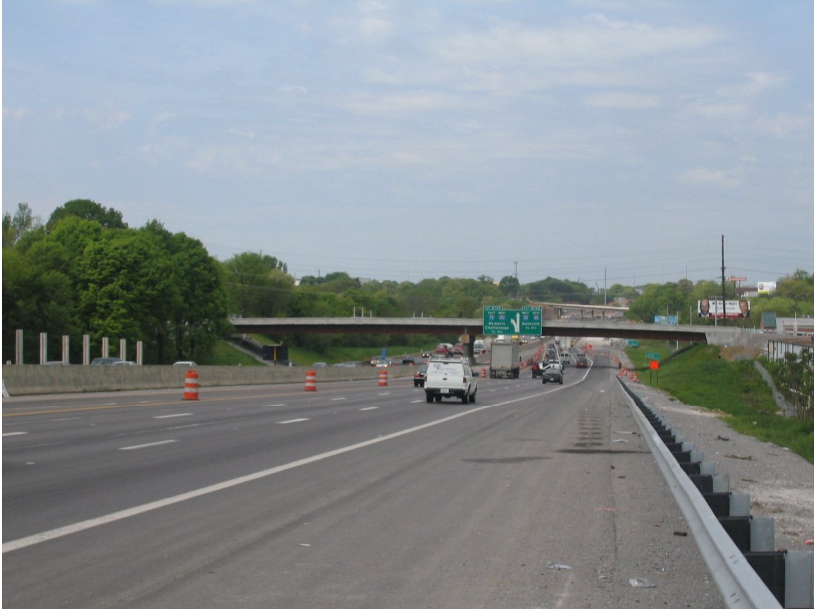
Figure A54: Photograph of Completed Massman Drive Bridge (View along I-40 looking west)
