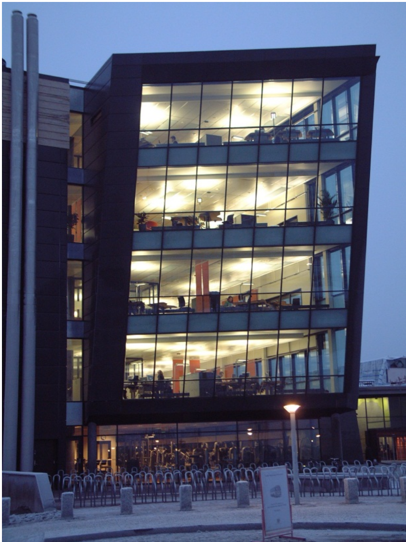
Figure 191. Telenor office building. Photo Jan Draplos
