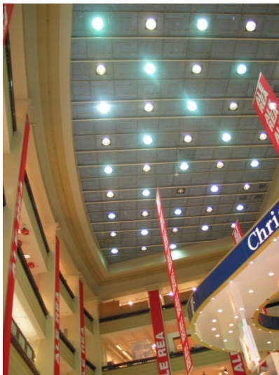
Figure 248. Lamp luminaires integrated in the glass panels. Photo Julle Oksanen
