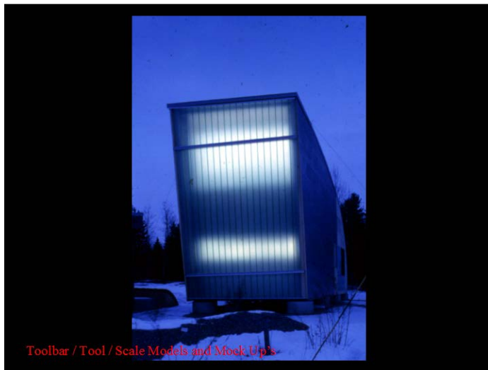
Figure 302. KIASMA Mock' Up 1:2 built from floors 4 and 5. Photo Timo Kiukkola
