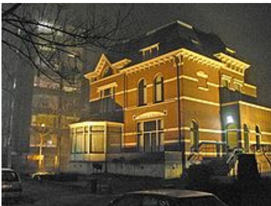
Figure 15. Facade lighting ( www.darksky.org ).
