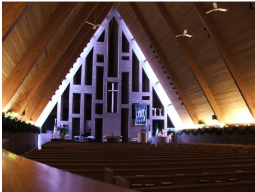
Figure 235. Clerestory labeled a skylight. Photo Richard Kelso
