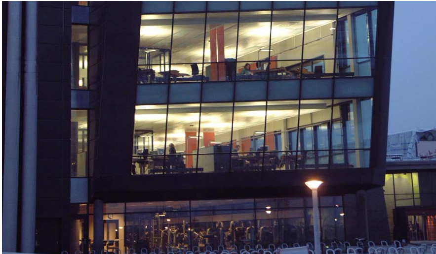
Figure 192. Telenor office building. Photo Jan Draplos
