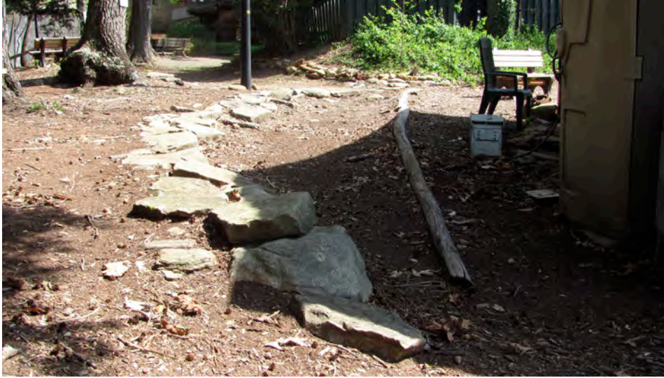
Figure 5.11 - Make-shift level spreader in downtown Montreal*
