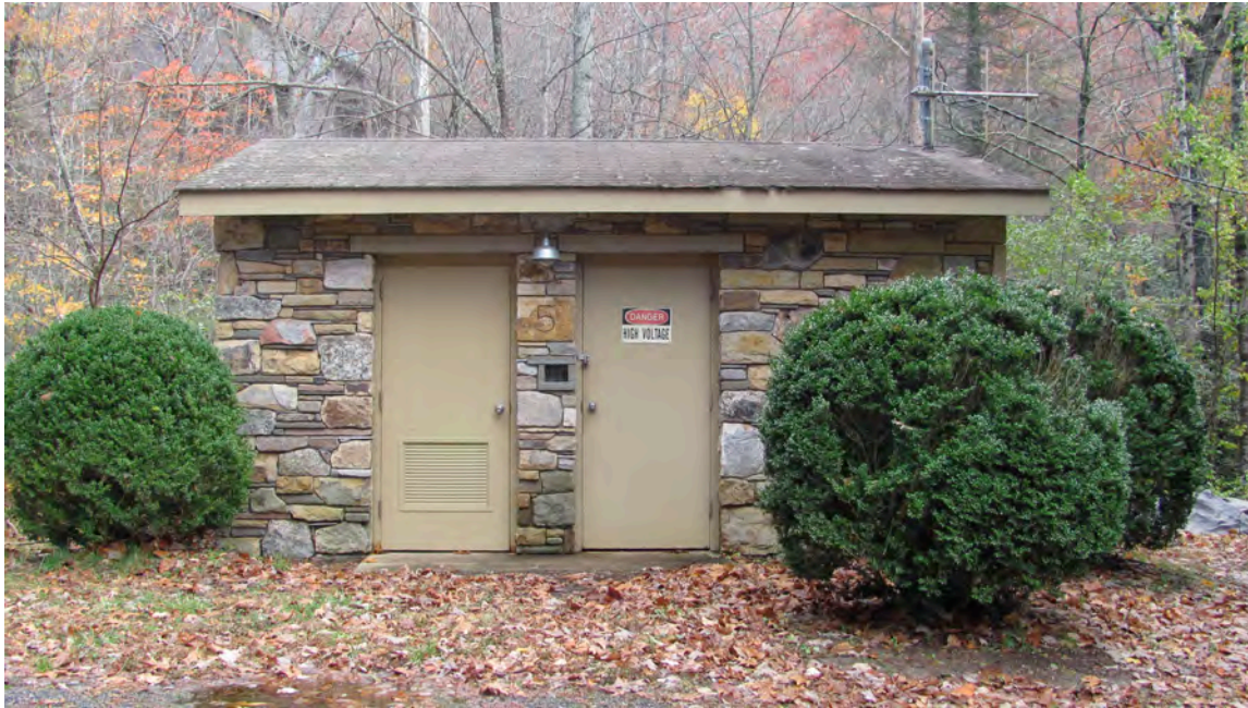
Figure 3 - Well Pump House and Water Filtration Facility #1-A in Montreat*
