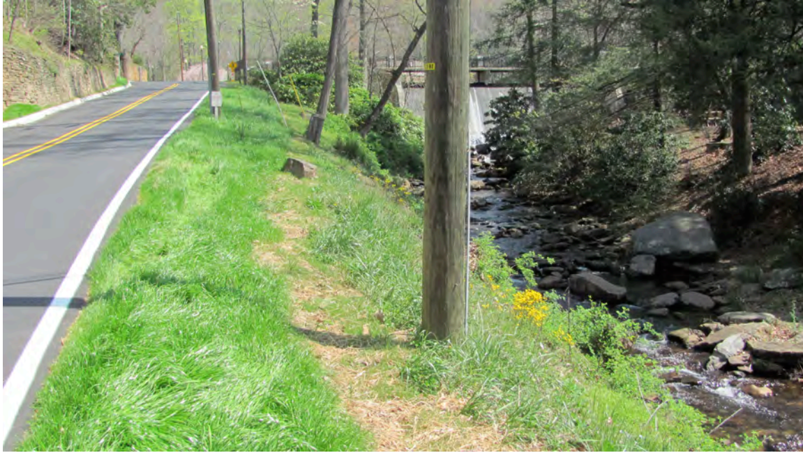
Figure 5.5 - Site for proposed roadside swale*
