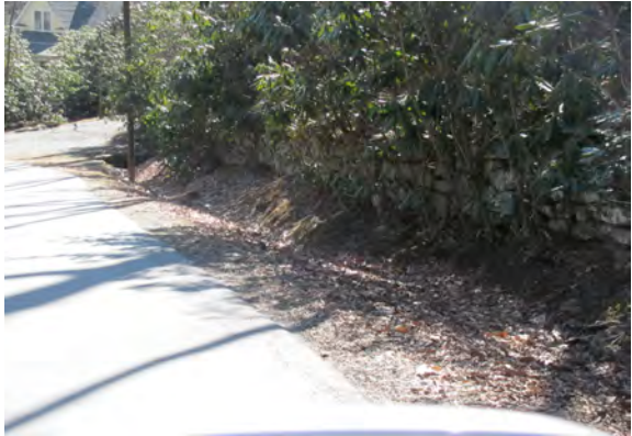
Figure 5.6 - Site for proposed roadside swale*
