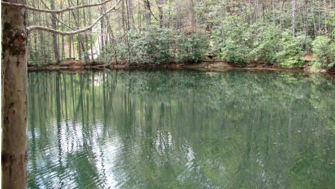
Figure 5.13 - Montreat town reservoir*
