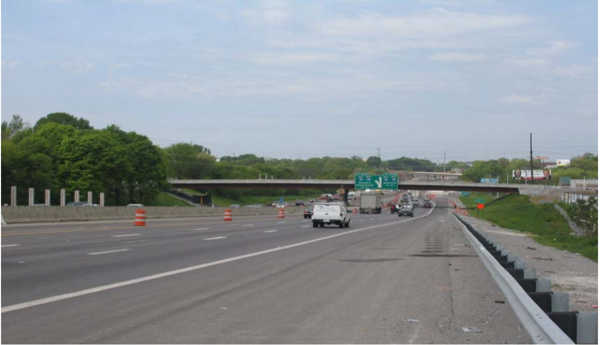
Figure 2.1: Photograph of Massman Drive Bridge Elevation Looking West
