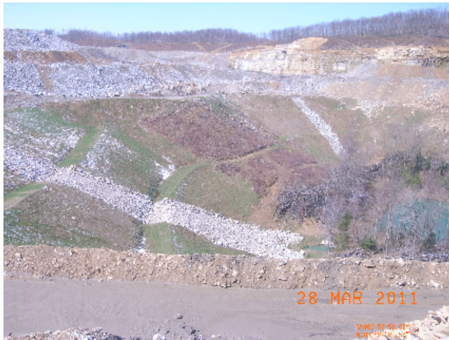
Figure 28: Site Photo D - Brown ground between them is original ground, not disturbed/mined. There is a small sump at the Toe of VF 3, not required or on the map, done as a sediment trap. Pond 2 is lower on right. The trees from the clear-cutting are windrowed along the lower edge of the permit boundary. The jumbled/piled material on the top of the valley fill (above the trucks on the left) is the reclamation of the cross hatched area on the ridge between valley fill 2 & 3. The structure in the foreground is a constructed sediment ditch on the Clarion level. The valley fills are benched off at 100' levels both have 3 benches. They also have their center drains constructed and rip-rapped (Curry).
