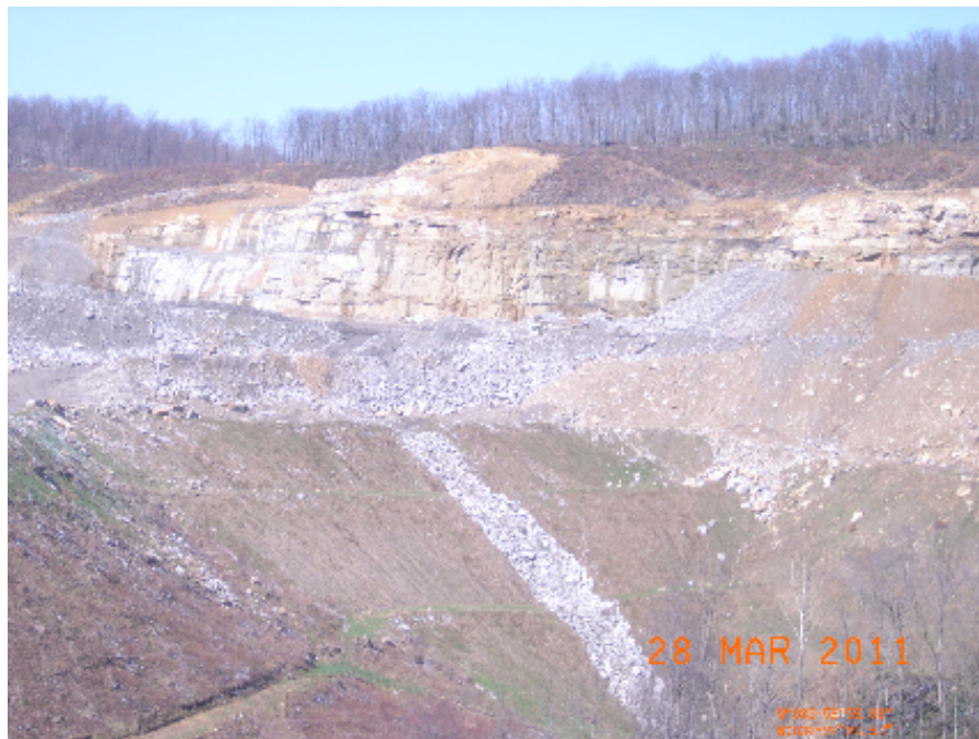
Figure 27: Site Photo C - This section of wall will be left open (not backfilled). CONSOL (Fola) is going to put in a deep mine face-up here (Curry).
