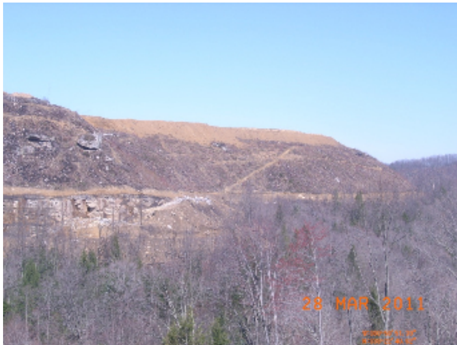
Figure 31: Site Photo G - Shows highwall development along the Lower Kittanning level which will become a contour cut around the ridge. This contour cut will become a buffer and will temporarily divert water back toward head of the hollow during the mining (Curry).
