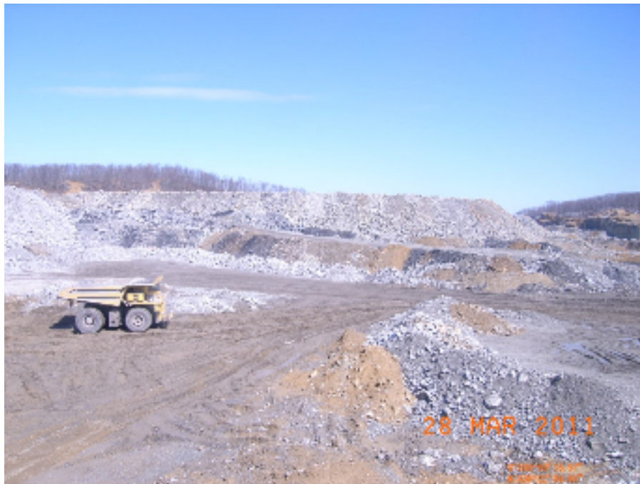
Figure 33: Site Photo I - The spoil piled up in the background was generated when the ridge was mined and will stay there until later. The trucks are hauling from active mine sites and reclaiming the highwall and this ridge. After the other sites are mined (no more spoil) or if the other sites continue and this site is near reclaimed, then the prepositioned spoil will be moved back to finish the reclamation. The piles of brown are topsoil stockpiles (Curry).
