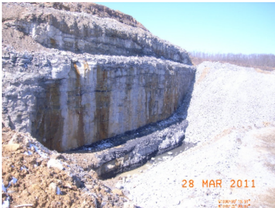
Figure 32: Site Photo H - Highwall at the permit boundary across the bridge between VF 2 & 3. The spoil is coming from the mining in previous pictures. This wall is on the black line at the SE end of the cross hatched ridge between the VF's. The material is being dumped by truck and gets ramped up to the top of the highwall. This minimizes the amount of shoving by bulldozer (Curry).
