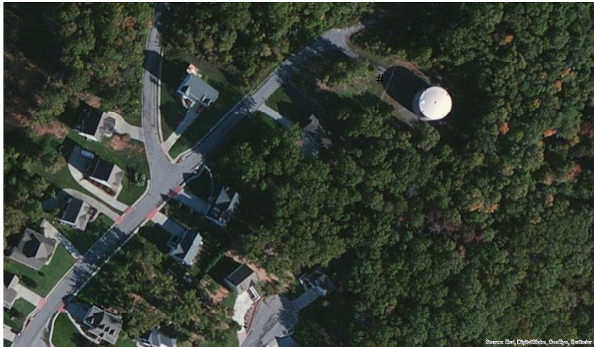
Figure 39. Example of Distributed Storage Testing Location in Cleveland, TN.
