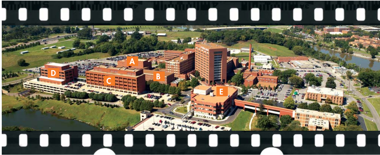
Medical buildings A (1990), B (1967), C (1985), D (2003) and E (2004).
