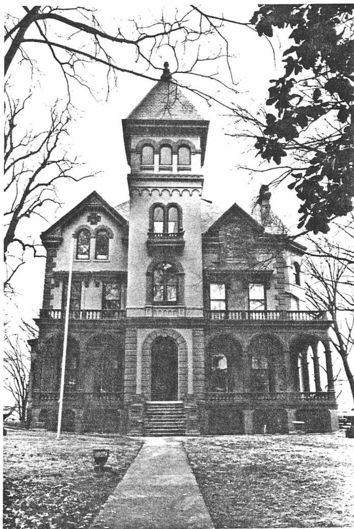
Figure 39. Mallory-Neely House as it appears today with J. C. Neely's post-1890 additions grafted on top of Kirtland's c. 1852 Italianate villa.
