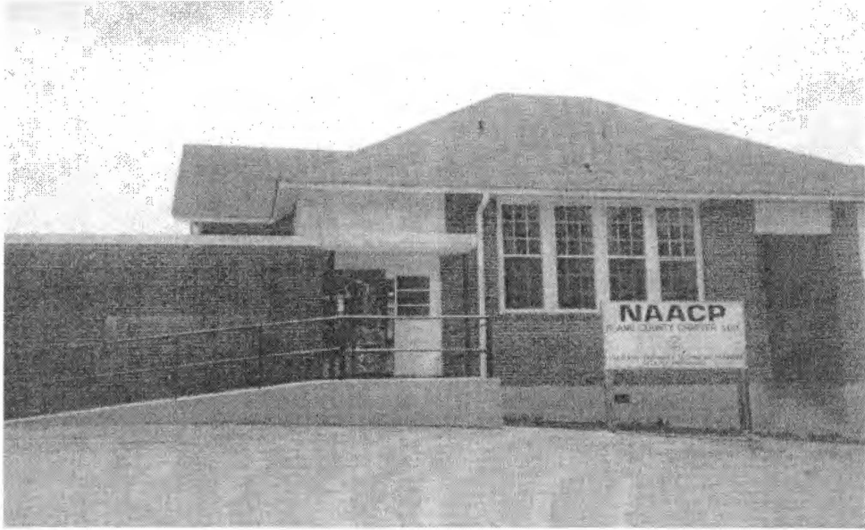
Figure V-26. NAACP Building, Greenwood Neighborhood. Former Greenwood community school is now a local chapter of the NAACP. Margaret D. Foraker 2000.
