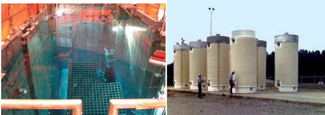
Figure 1: On the left is a spent fuel pool filled with spent fuel assembly racks [5]. On the right are vertical storage overpacks storing dry canisters [6]
