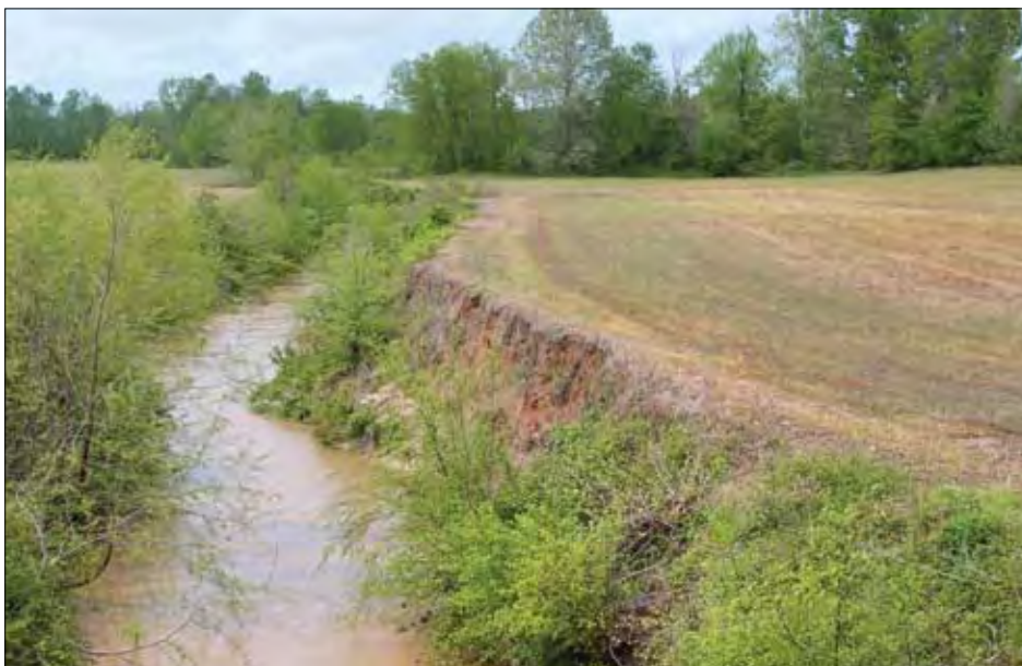
Fig. 2.28 Buffers established adjacent to drainages can prevent sediment flow and provide critical habitat that can support many wildlife species and help increase wildlife populations. A native grass buffer is much needed along the edge of this drainage ditch.
