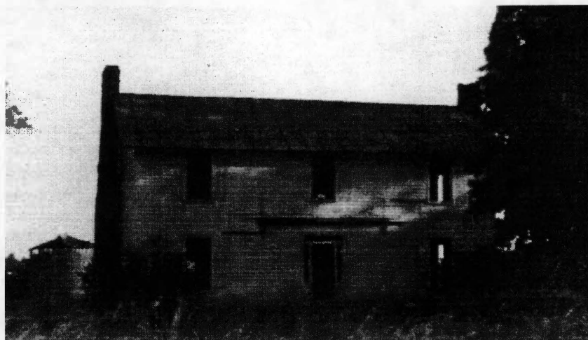
Plate 5.2. Tipton/Dixon House in 1976, Prior to Demolition by TVA (photograph by L.Lane).
