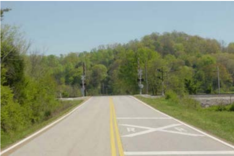
Figure 4: CSX At-grade Railroad Crossing, looking east
