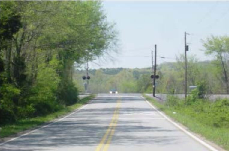
Figure 5: CSX At-grade Railroad Crossing, looking west
