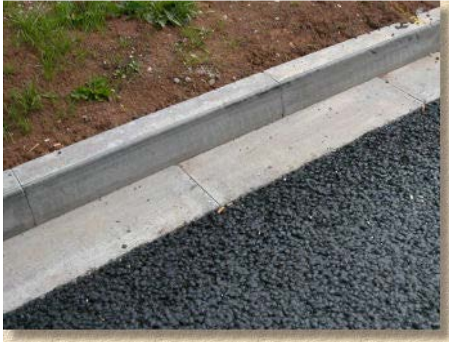
Figure 4.2: Barrier Type Curb
