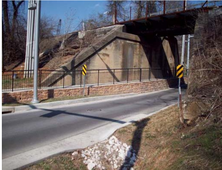
Figure 5.1: Blount Ave. Elevated Sidewalk (Southern Constructors, Inc. 2016)
