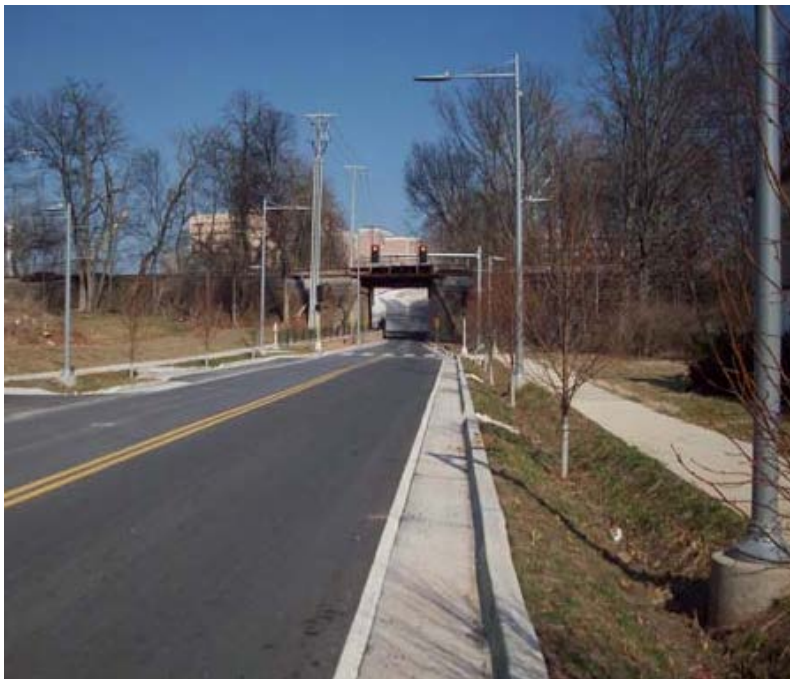
Figure 5.2: Blount Ave Signalized Approach (Southern Constructors, Inc. 2016)
