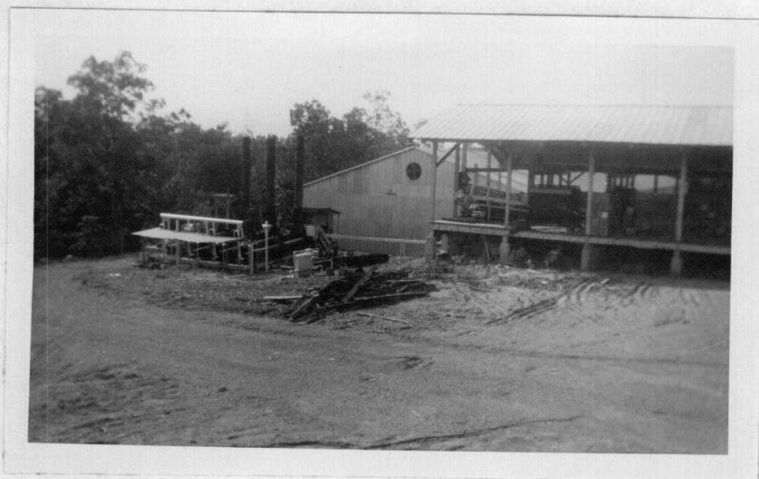
Figure 81. The steam boilers and unloading docks of the Monticello Canning Company plant.
