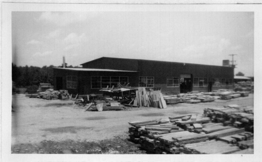
Figure 65. The fabrication mill of the Crab Orchard Stone Company; a stonecutter's bench is in the foreground.
