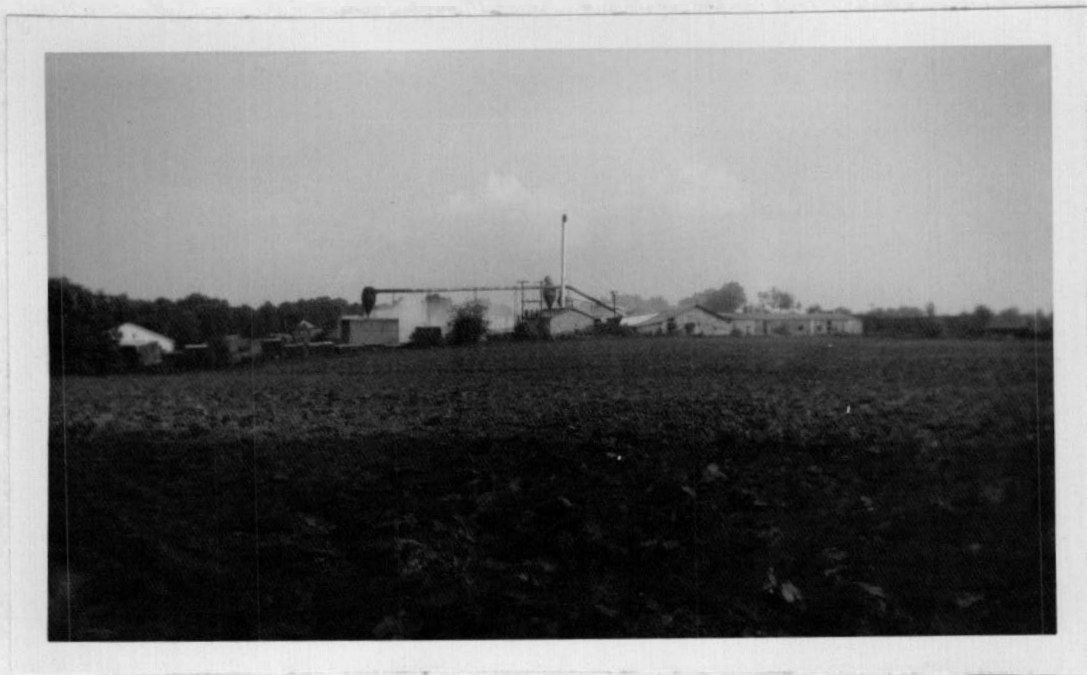
Figure 79. The Crossville Lumber Company mill.
