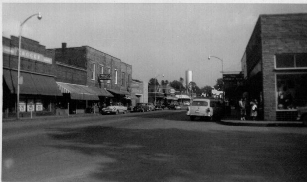
Figure 18. The principal street in Crossville's business district.
