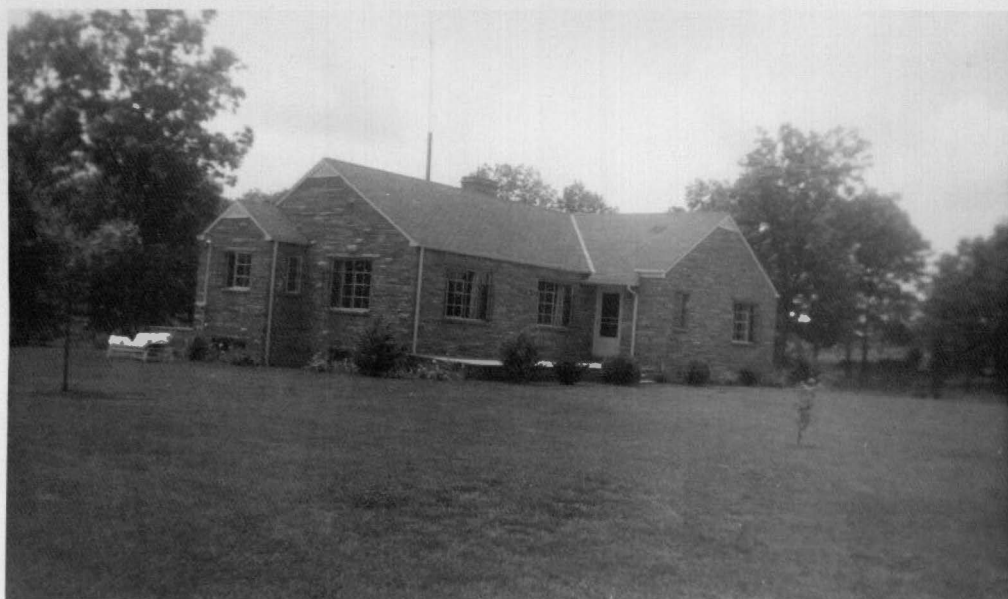
Figure 62. A heavy strip rubble sandstone house.
