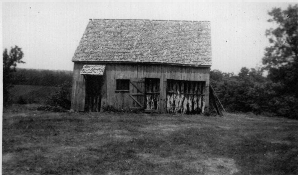
Figure 36. A barn filled with Burley tobacco for air curing on a farm in the Cumberland Homesteads area.
