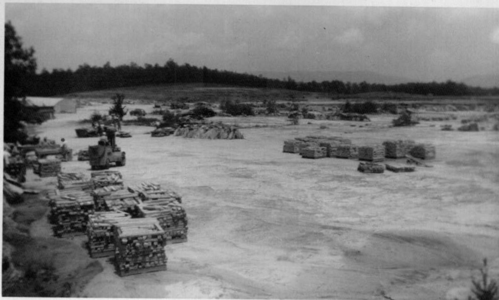
Figure 60. The fifty-acre sandstone quarry of the Crab Orchard Stone Company.
