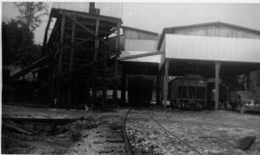
Figure 54. The coal loading tippel for the mine at Isoline.
