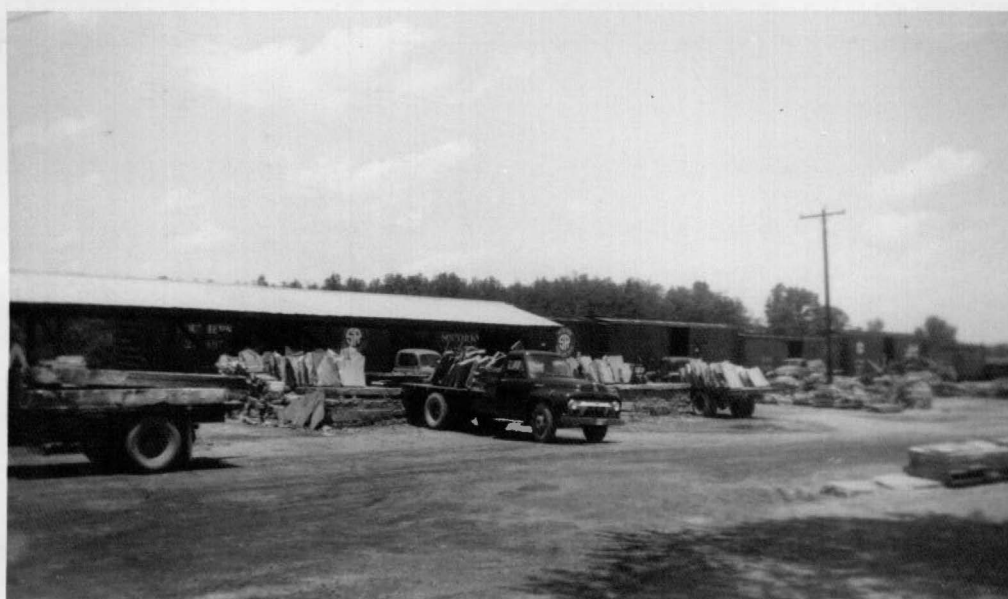
Figure 66. The loading dock of the Crab Orchard Stone Company at Dorton a few miles east of Crossville on the Tennessee Central Railroad.
