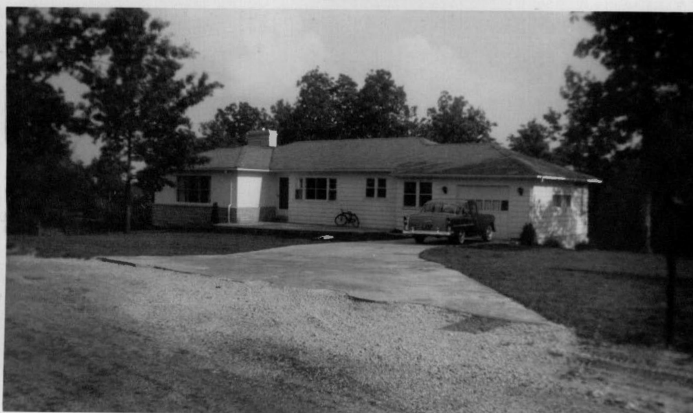
Figure 14. A typical home in Volunteer Heights, a modern subdivision south of the Crossville city limits.
