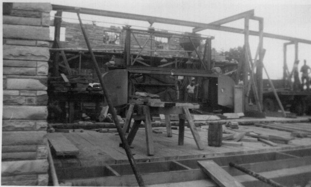
Figure 63. A hydraulic guillotine for breaking sandstone flags into strip rubble.
