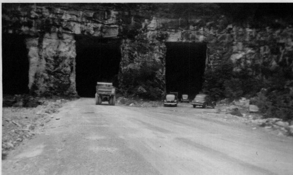
Figure 68. Entrance to the Southern States Lime Corporation mine at Crab Orchard.
