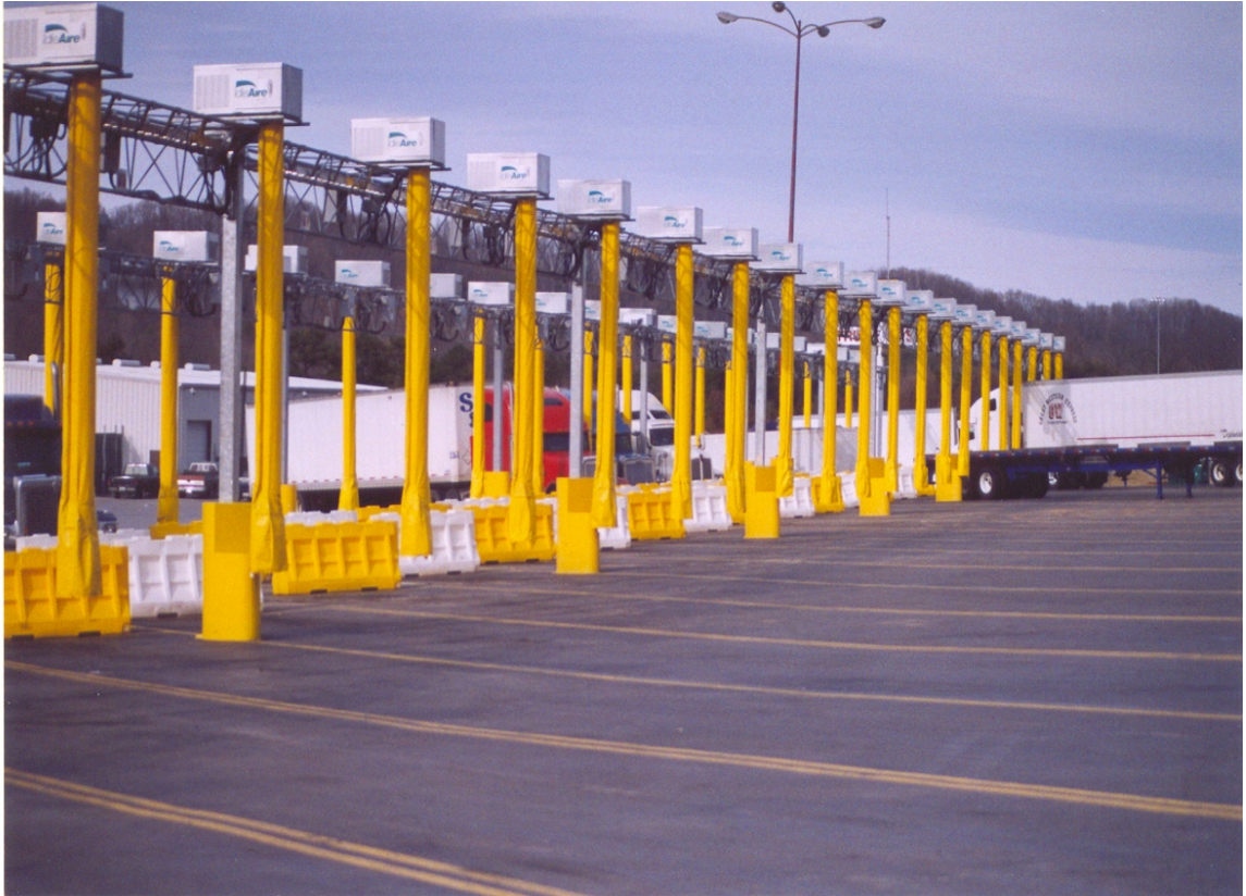
Figure 1.1 IdleAire Electrification Units at Petro Truck Travel Center
