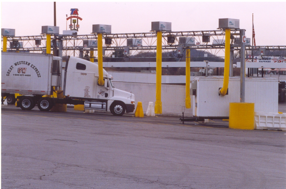
Figure 3.3 A Truck and One of the Monitoring Trailers Connected to IdleAire Electrification Units
