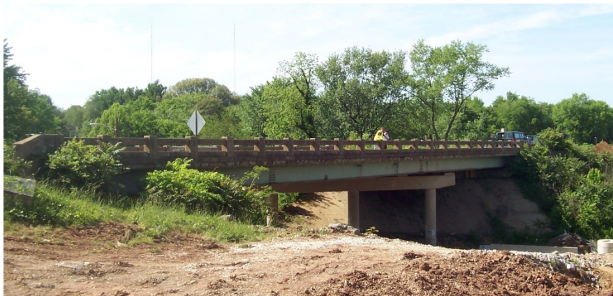
Figure 3.8. Photo of the I-40 westbound bridge over 4th Avenue
