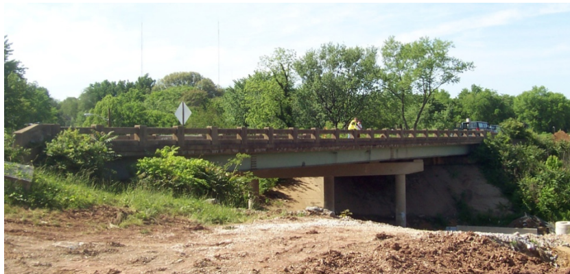
Figure 2.10. Photo of the I-40 westbound bridge over 4th Avenue
