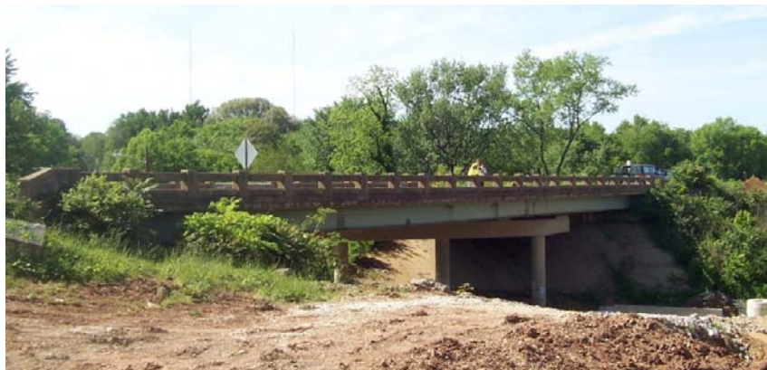
Figure 4.1. Photo of the I-40 westbound bridge over 4th Avenue
