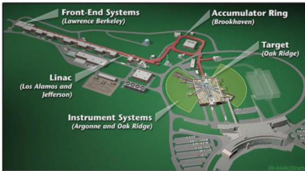
Figure 1.1 Spallation Neutron Source conceptual layout. The SNS was built by a partnership of six U.S. Department of Energy laboratories. [3]
