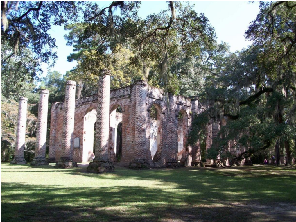
Figure 6-23. Ruins of Prince William's Parish Church. Columns are at the west entrance of the church. (Photo by the author).
