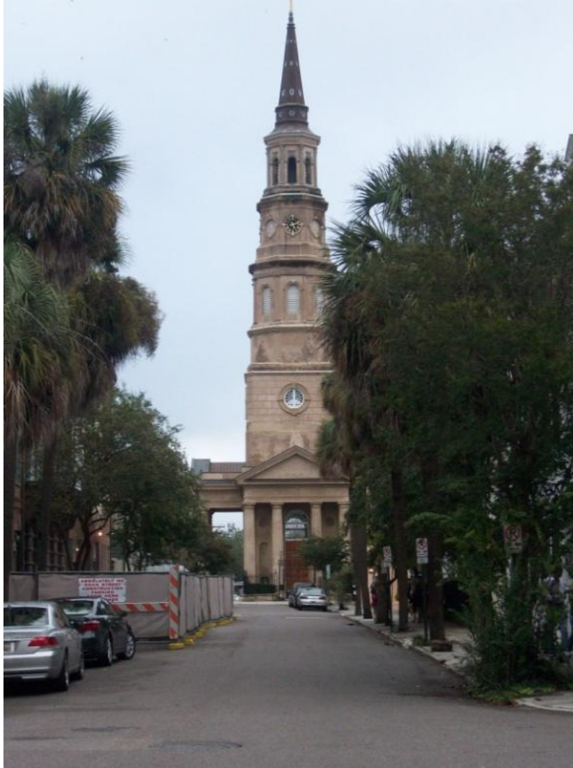
Figure 6-8. St. Phillip's Church. This ca. 1832 church was constructed so that its western portico still sat in the middle of Church Street. (Photo by the author).
