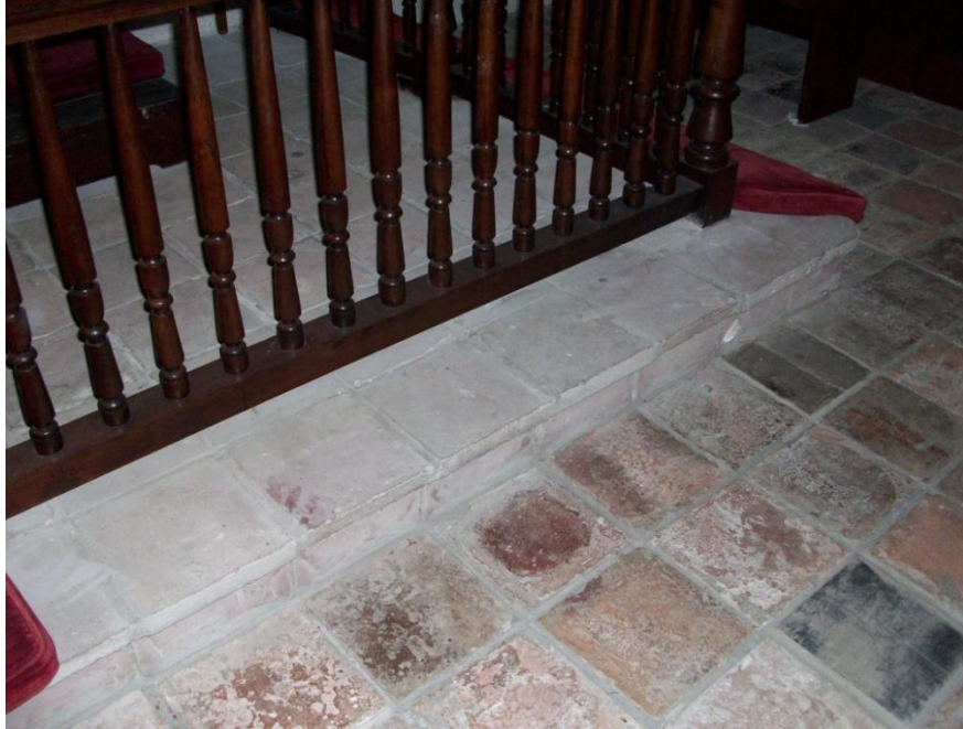
Figure 5-12. Communion rail at Strawberry Chapel. Cushion was removed from photograph to show brick pavers underneath. (Photo by the author).
