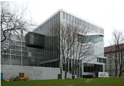
Netherlandy in Germany
