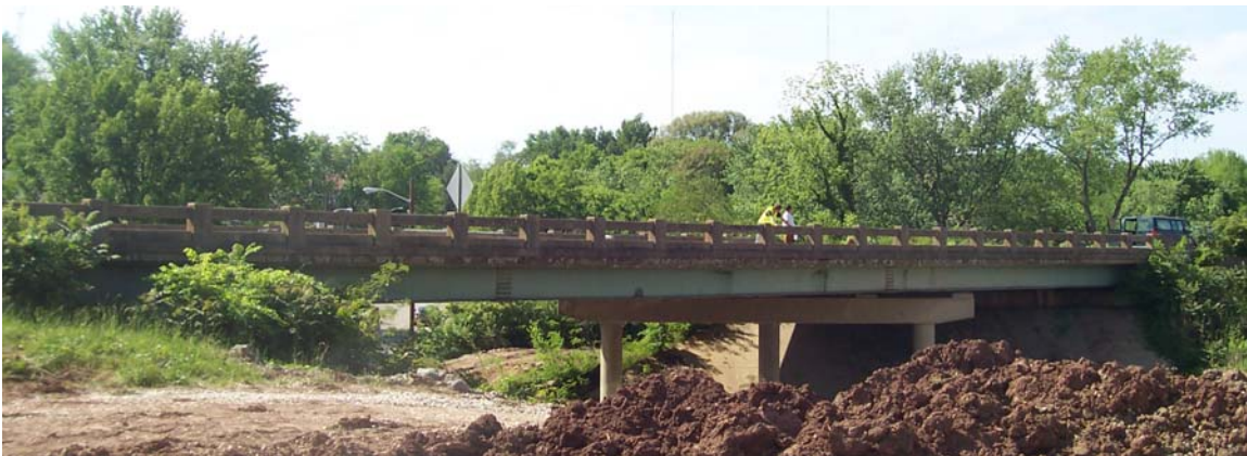
Figure 6.1. I-40 westbound over 4 th Avenue (47I00400066)
