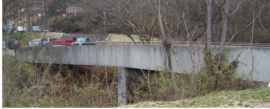
Figure 3.5. Test bridge at the University of Tennessee
