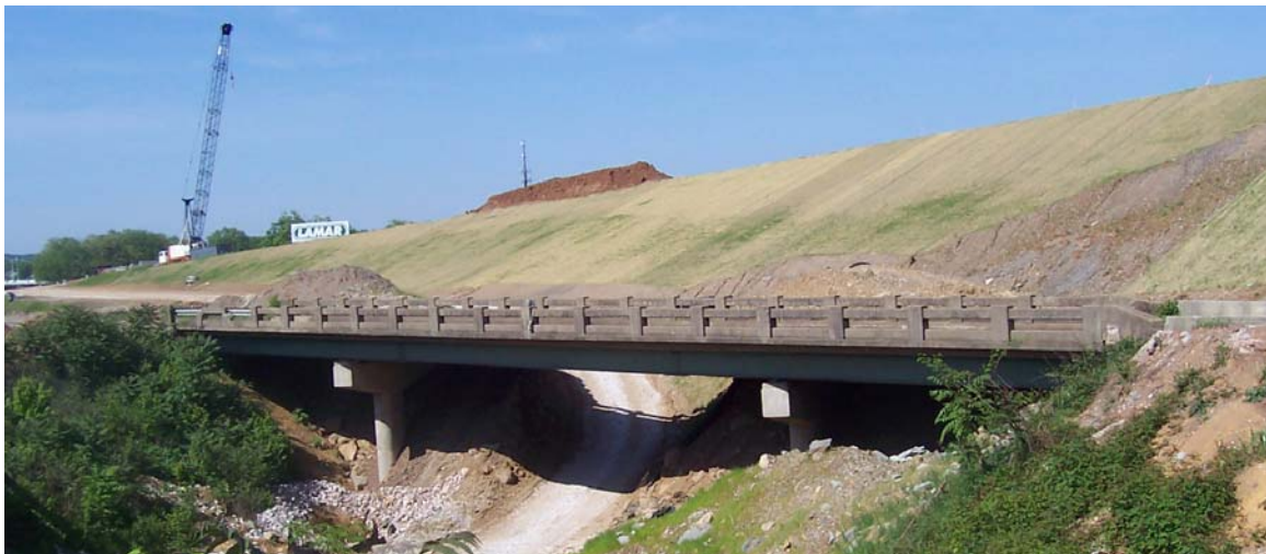
Figure 4.1. Entrance ramp to James White Parkway (47SR1580031)
