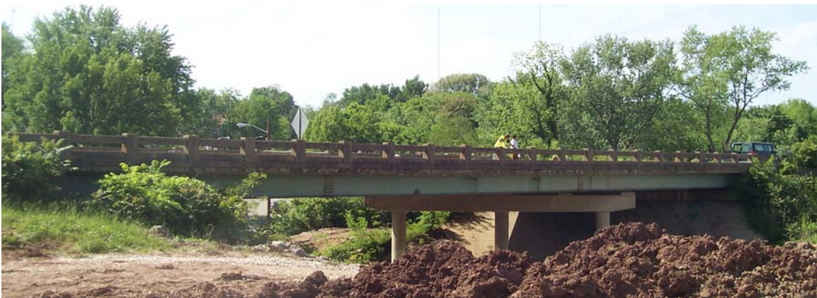
Figure 5.1. I-40 westbound over 4 th Avenue (47I00400066)
