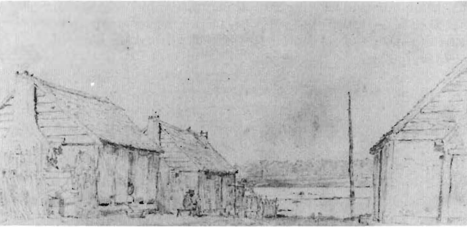
Slave cottages west of Charleston, from Hall, B. MSS no. 65, Manuscripts Department, Lilly Library, Indiana University, Bloomington, Indiana. Capt. Basil Hall (1788–1844) was the British author of Travels in North America in the Years 1827 and 1828 (London and Edinburgh, 1829).
