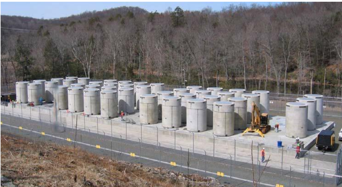
Figure 2: Spent fuel storage site at Connecticut Yankee Nuclear Power Plant [3]
