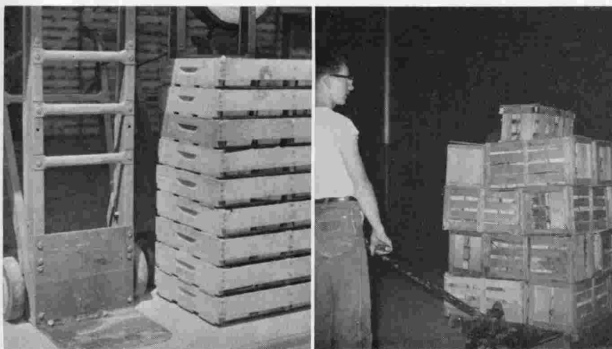
Figure 20. Hand truck (left) and dolly (right) used for transporting strawberries.
