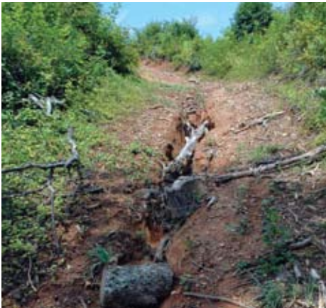
Fig. 12.5 This road was planted with orchardgrass in September after the logging operation was completed. Orchardgrass is a perennial cool-season grass and is relatively slow to establish. Precipitation through the fall and winter eroded this road before the orchardgrass could become established. The problem with this erosion, however, was not related to orchardgrass, but improper road construction. No planting will hold soil together on a road coming straight down the hill. The bottom line is orchardgrass and tall fescue are not “cure-alls” to prevent erosion of forest roads. Sensible road construction and use of annual and “wildlife-friendly” perennials, as well as the seedbank, are much better solutions for managing woods roads after logging.
