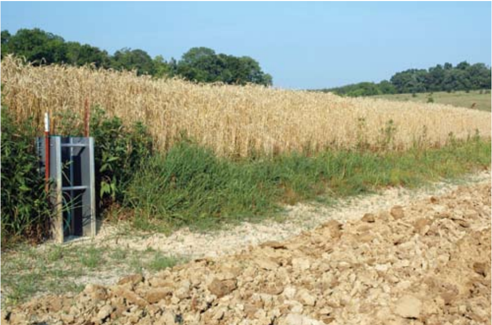
Fig. 11.2 A water-control structure allows the water level to be manipulated when fields are flooded.
