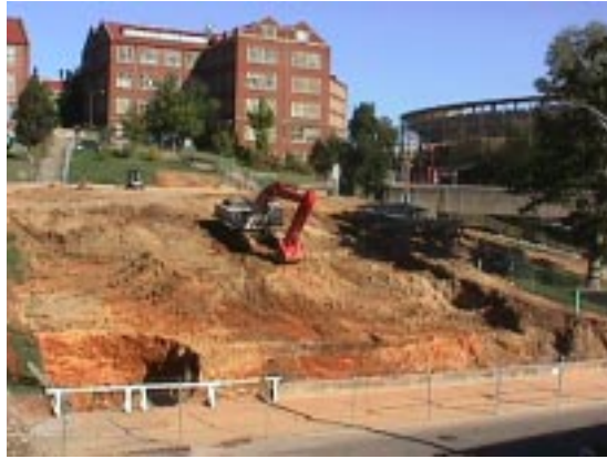
Excavation for Burchfiel Geography Building 10/23/98
