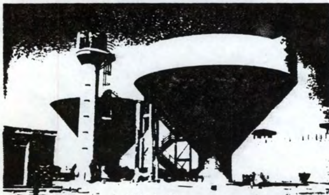
In conjunction with these two 51'-6" \emptyset lime softening Claricones, CBI Walker provided a Headtank/Trav Aerator assembly for the removal of \text{CO}_2 and
